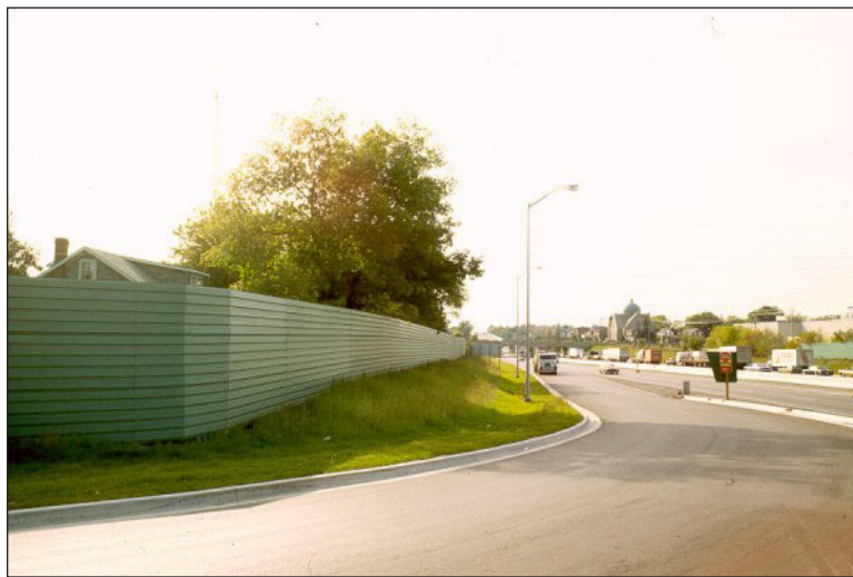
Figure 23 Wrap-Around Noise Barrier (Source: Fleming et al. 2000)
