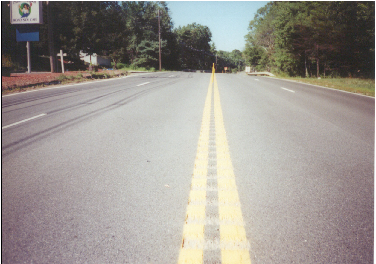
FIGURE 6. Centerline Rumble Strip on State Route 20 in Massachusetts.
