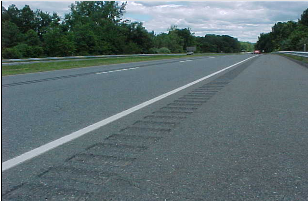
FIGURE 5. Linear Milled Shoulder Rumble Strips.
