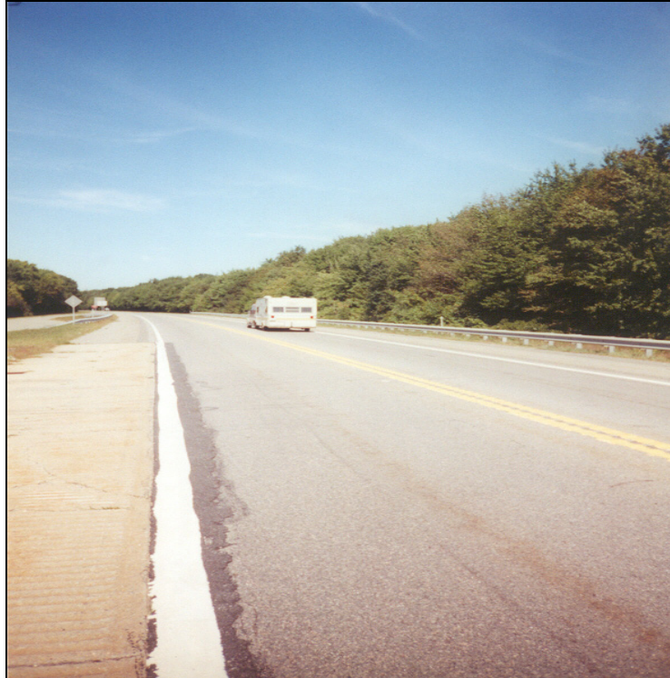
FIGURE 7. Centerline Rumble Strip on State Route 88 in Massachusetts.
