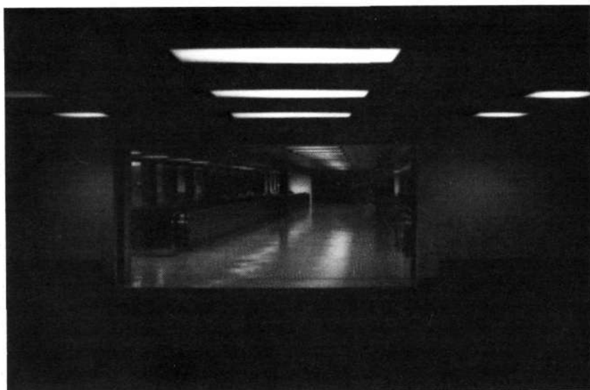
FIGURE 56. A moving walkway used in an enclosed pedestrian bridge connection between a multi-level parking structure and air terminal facilities at La Guardia Airport, New York, N.Y.
