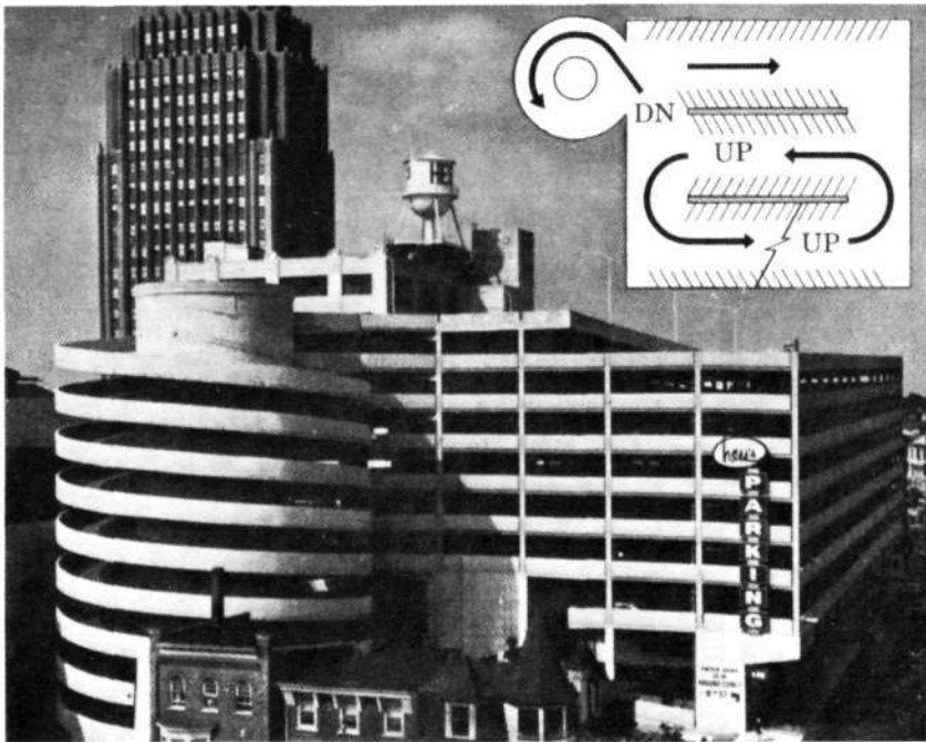
FIGURE 46. Helical ramps such as this one serving an 8-story, 750-car structure, can be used effectively for express exiting.
