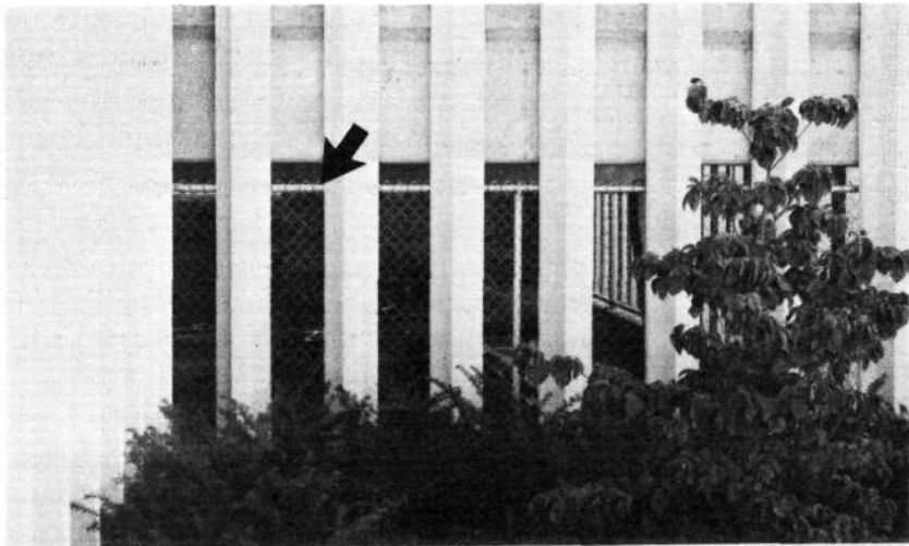
FIGURE 31. Chain-link fencing added to the ground-level of this garage prevents random pedestrian entry.
