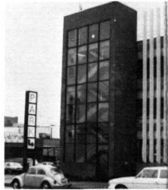
FIGURE 32. Where building codes permit, transparent stairwell enclosures can improve security.
