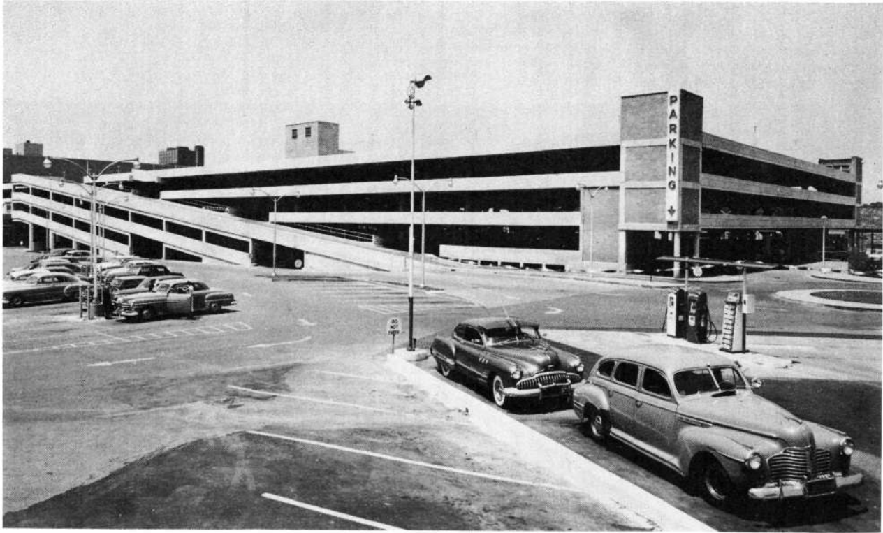
FIGURE IX-1. Outside ramp, Hecht Company garage, Arlington, Virginia.
