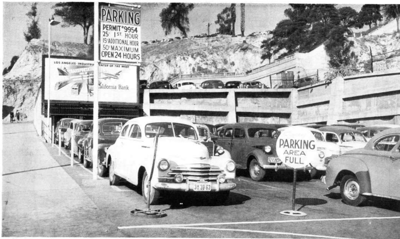
FIGURE 3. This Sign Gives All Information Required by the Los Angeles Ordinance for Parking Lot Signs.
