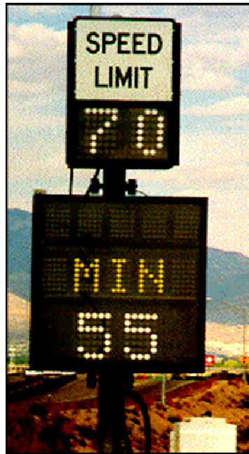
Figure 8-10: Variable Speed Limit Sign.
