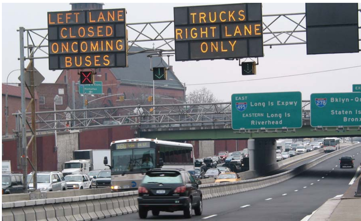
Figure 8-1: Example of Managed Lanes
