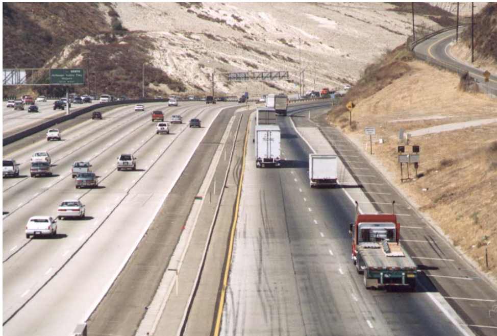
Figure 8-4: I-5 Truck Bypass, Los Angeles
