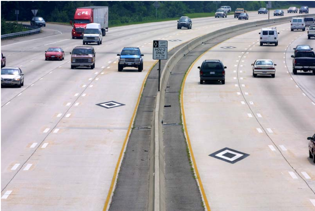
Figure 9-3: Example of Concurrent Flow Lane (Courtesy Virginia Department of Transportation)
