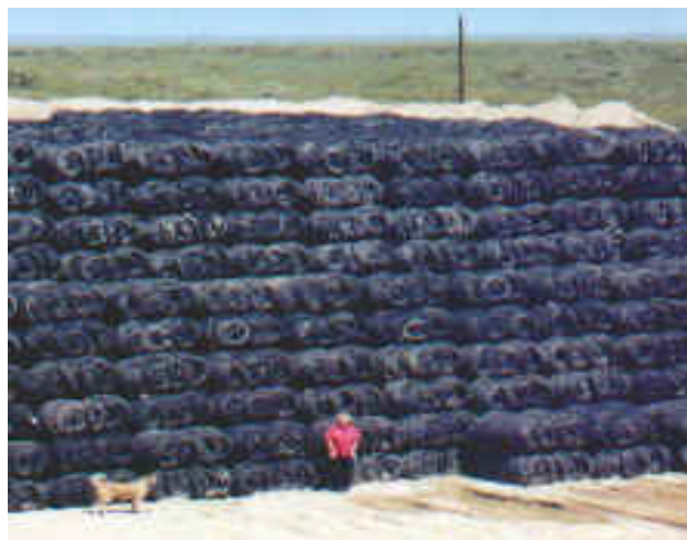
Figure 5.3. Stacked tire bales, e.g., to form the impact face of a rockfall barrier (Encore Systems, 2004)
