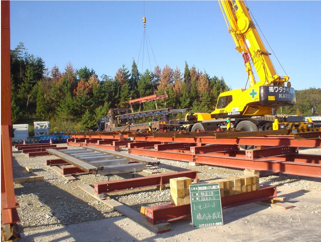
Figure 70: Guideway Section Staging for Transport Over the Guideway
