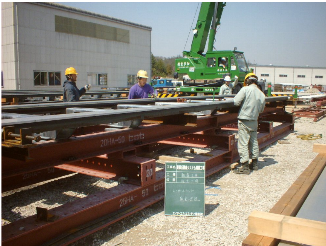
Figure 69: Levitation Rail Section Assembly Prior to Installation
