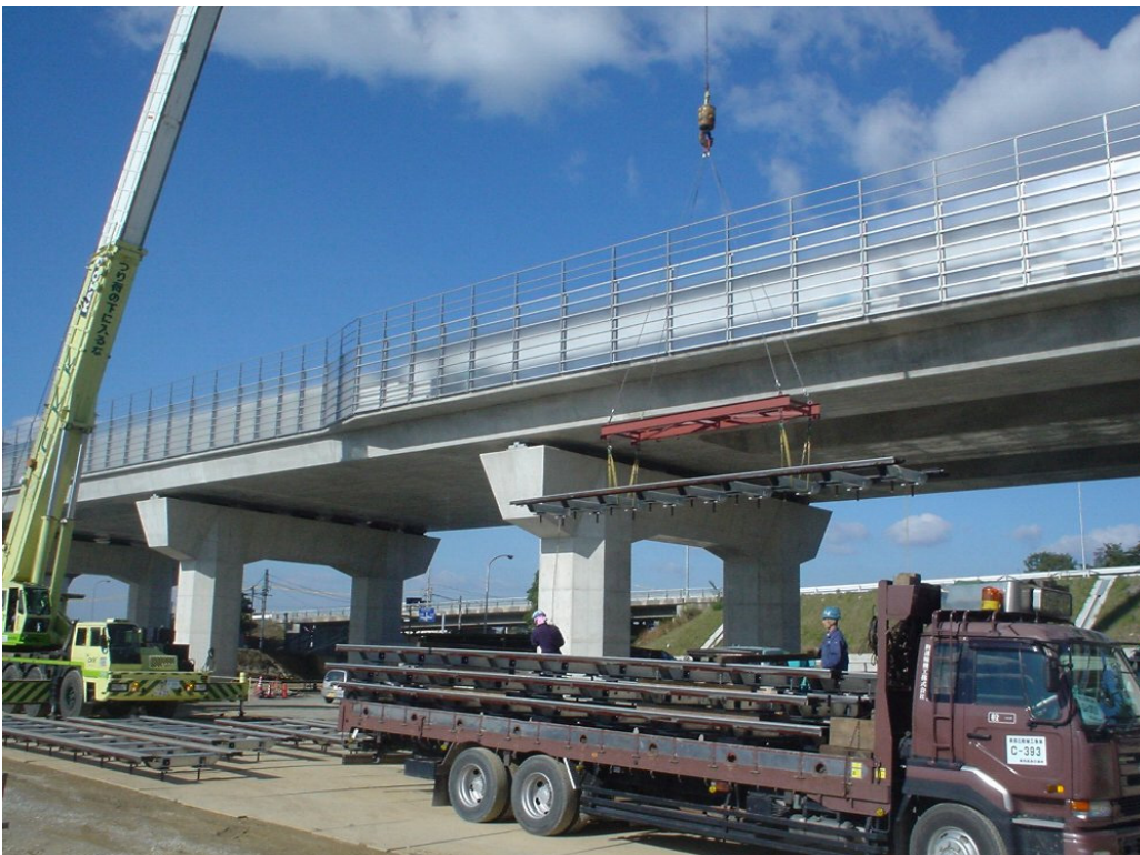
Figure 71: Guideway Sections Ready for Transport on the Guideway
