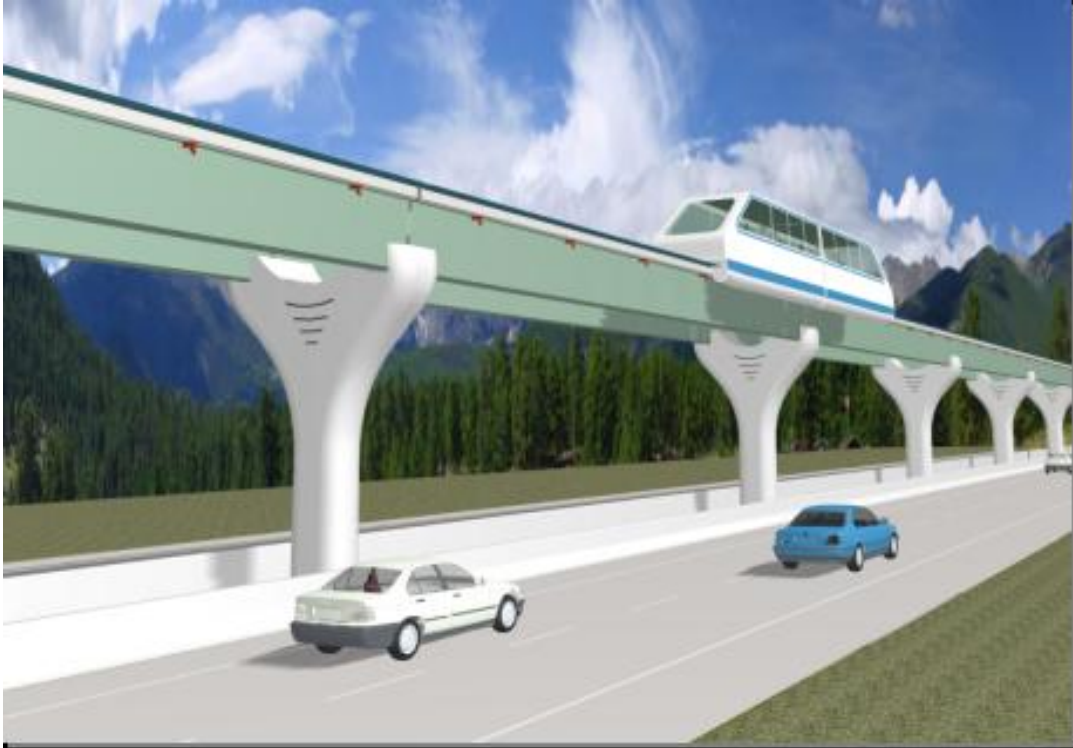
Figure A-10: Concept B: Rendering of Steel Box Girder Guideway
