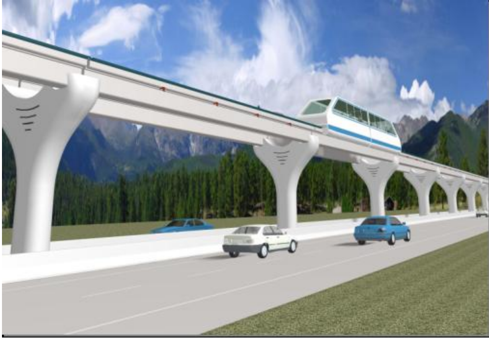
Figure A-9: Concept A: Rendering of Concrete U-Girder Guideway
