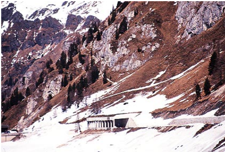
Figure B-32: Avalanche shed located in the Swiss Alps
