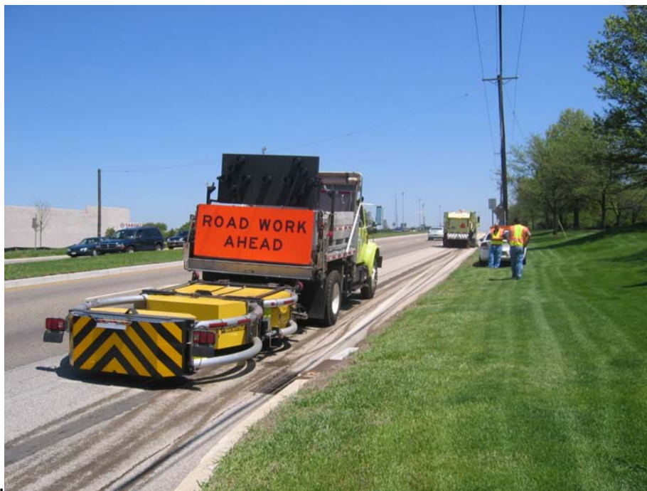
Figure 8 Shoulder Sweeping Operation
