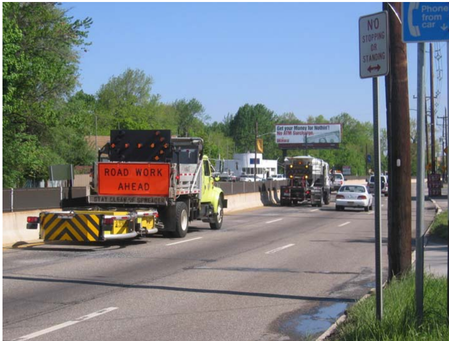
Figure 7 Pothole Patching Operation.
