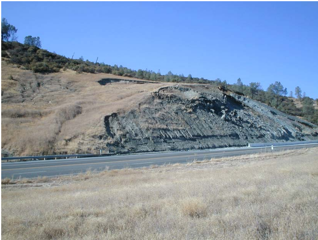
Figure 9 – Landslide on cut slope on State Route 20 in Colusa County
