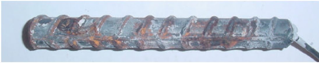
FIGURE 3.13: Conventional N3 anode bar after removal of mortar, at 15 weeks
