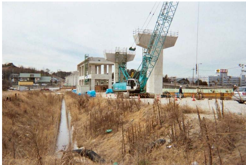
Figure 10. Columns Under Construction
