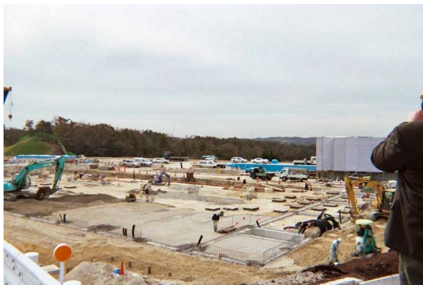
Figure 11. Maintenance Depot Under Construction
