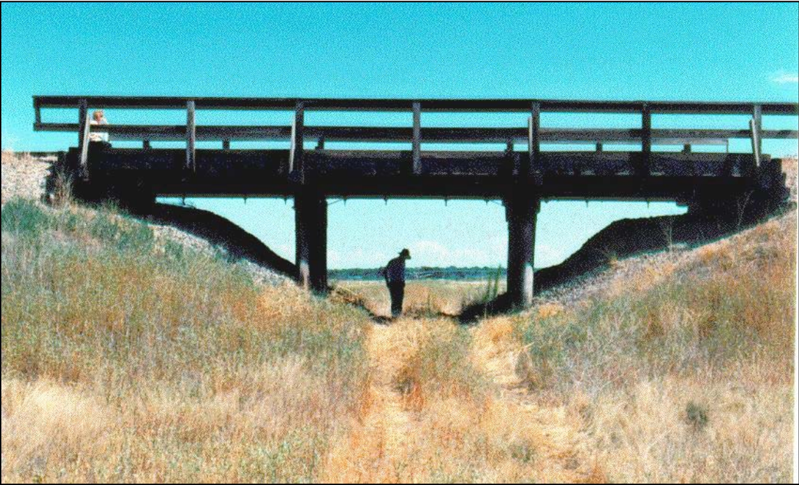
FIGURE 1. Bridge No. 101, View from West Side of Bridge
