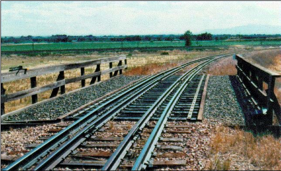
FIGURE 2. Bridge No. 101, View from North End of Bridge
