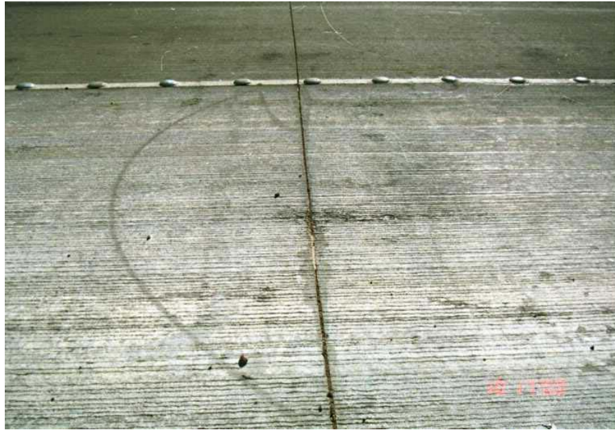
Figure 8. Surface Irregularity at a Transverse Joint
