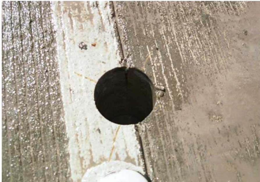
Figure 16. Core Hole - Longitudinal Joint
