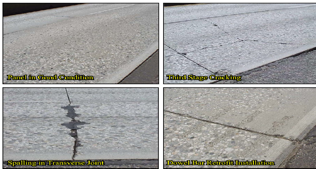
Figure 8. Pavement Condition - March 2001
