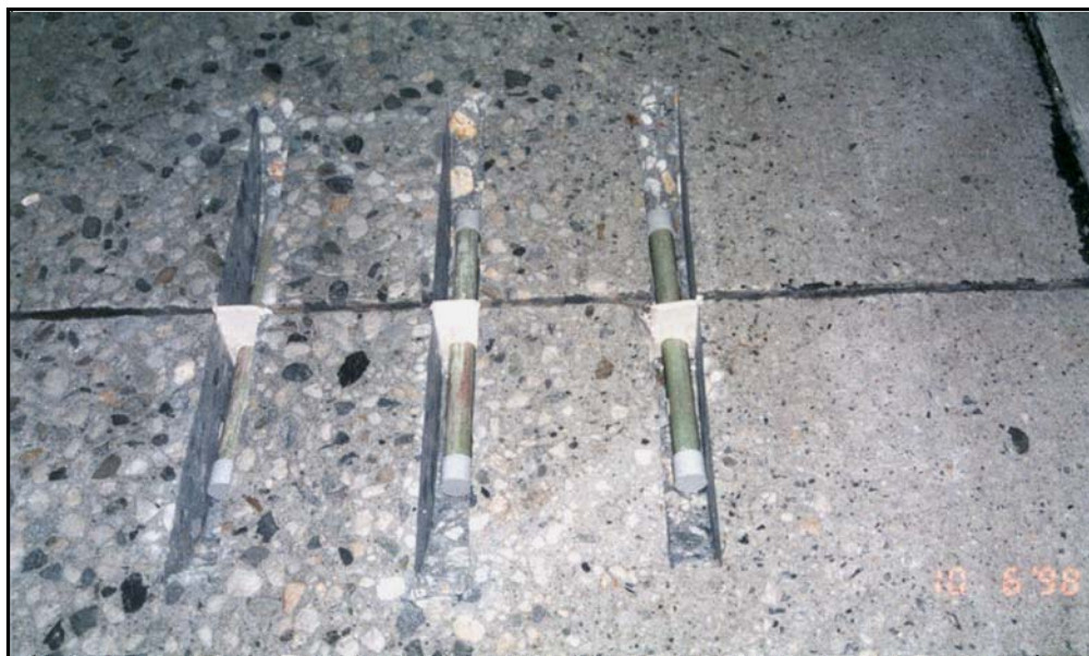
Figure 5. Dowel Bar Installation
