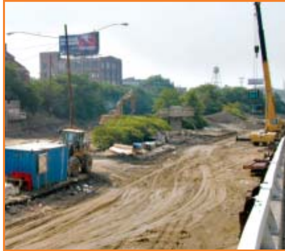
Figure 1. M-10 Under Full Closure
