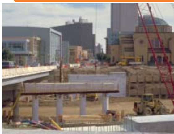
Figure 2. I-670 Under Full Closure
