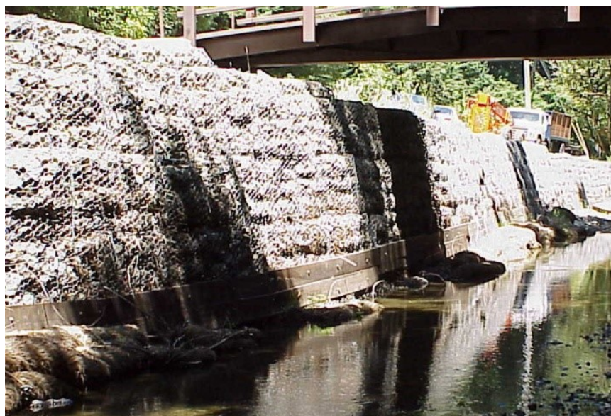
Gabion wall with timber facing to protect wires from abrasive flow.
