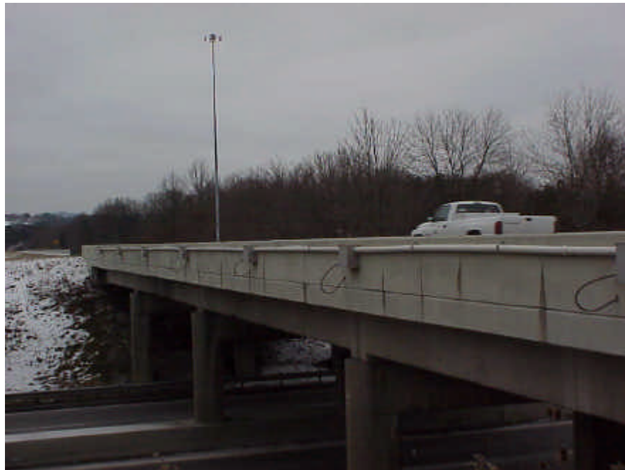
Figure 1. Spray System Mounted on Bridge
