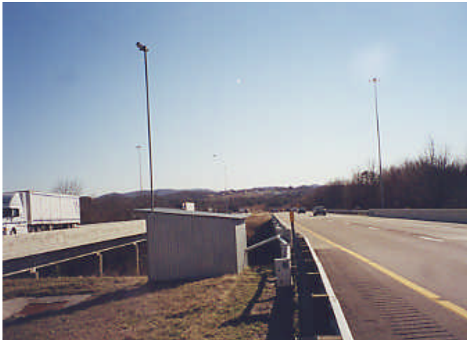
Figure 10. Twin Bridge Structures
