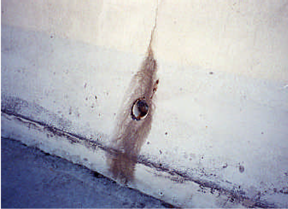
Figure 2. Spray Nozzle in Bridge Wall
