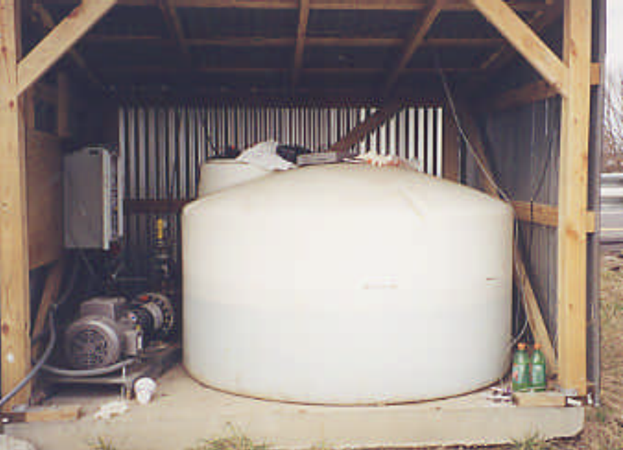
Figure 5. Inside Storage Building
