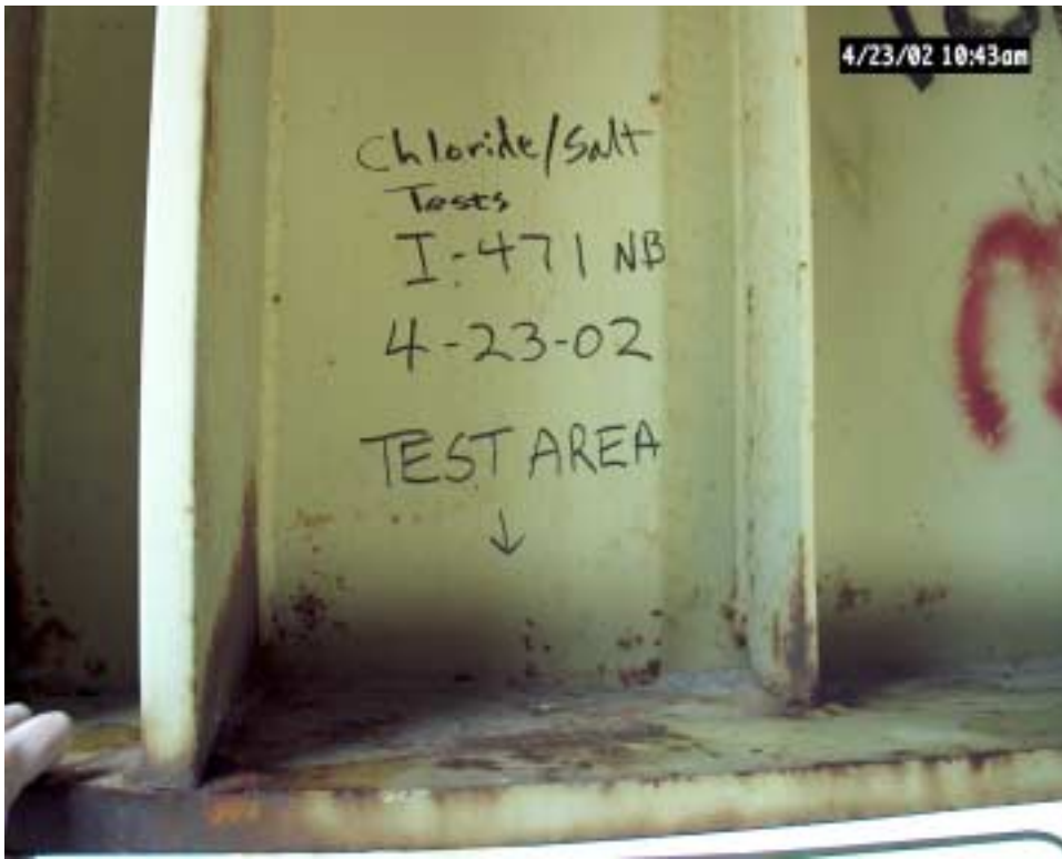
Figure 7 Test area power tool cleaned for collecting a sample on I-471N.
