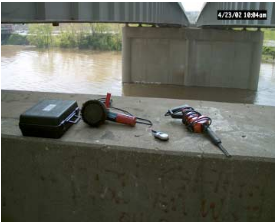
Figure 4 Power tools used in preparing a test area.
