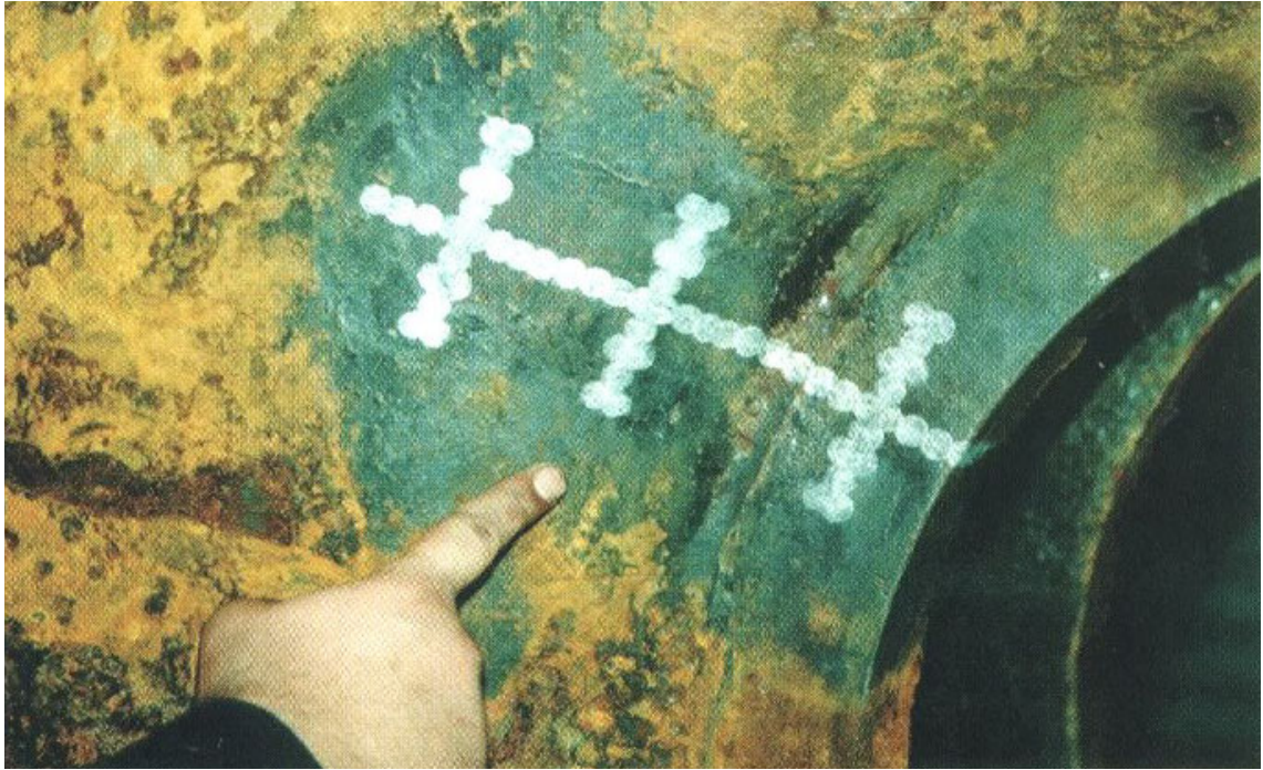
Figure 4.19 – Metal Stitching Completed – (Photo courtesy of Lock-N-Stitch Inc.)
