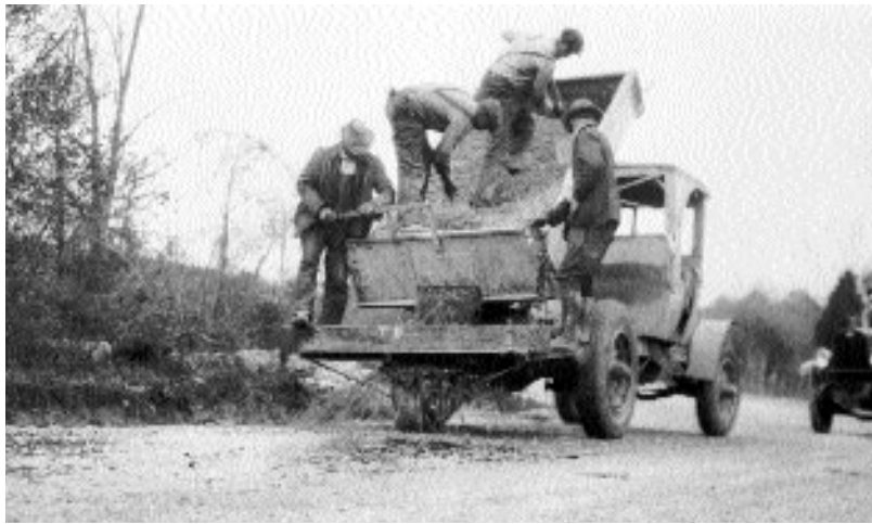
Chip spreader crew at work in Lynchburg District.
