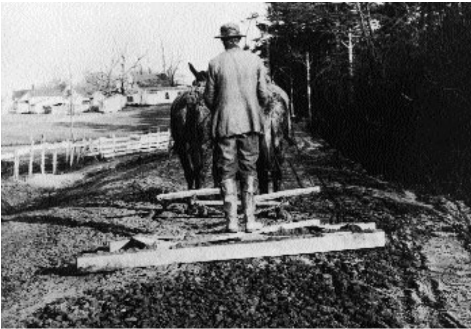
Inadequate funds for road maintenance meant it was crude and often neglected.
