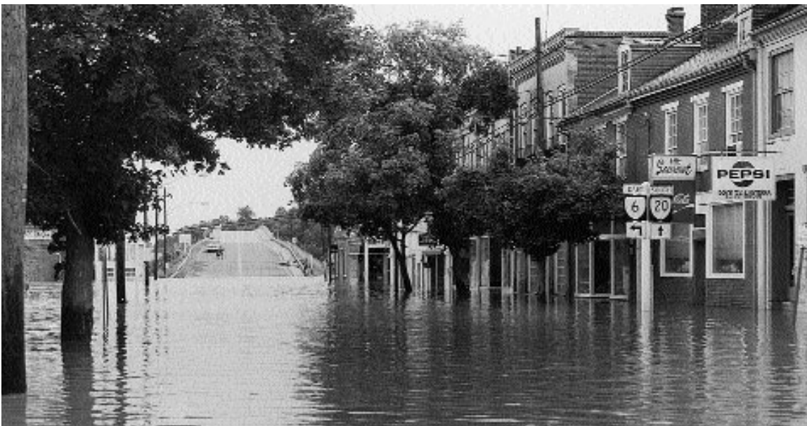
The flooding generated by Hurricane Camille resulted in the most devastating damage ever inflicted by nature on the state's highway system, as seen in part in this photo of Scottsville.
