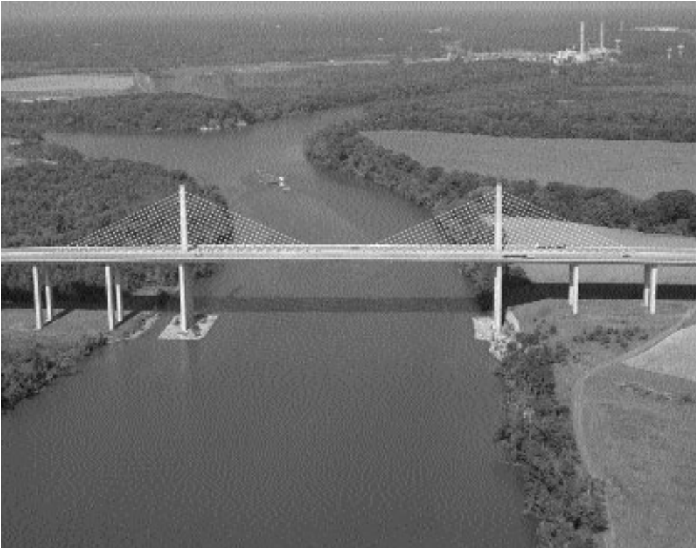
The I-295 cable-stayed bridge is one of few like it in the U.S. today. It crosses the James River south of Richmond between Varina and Enon.
