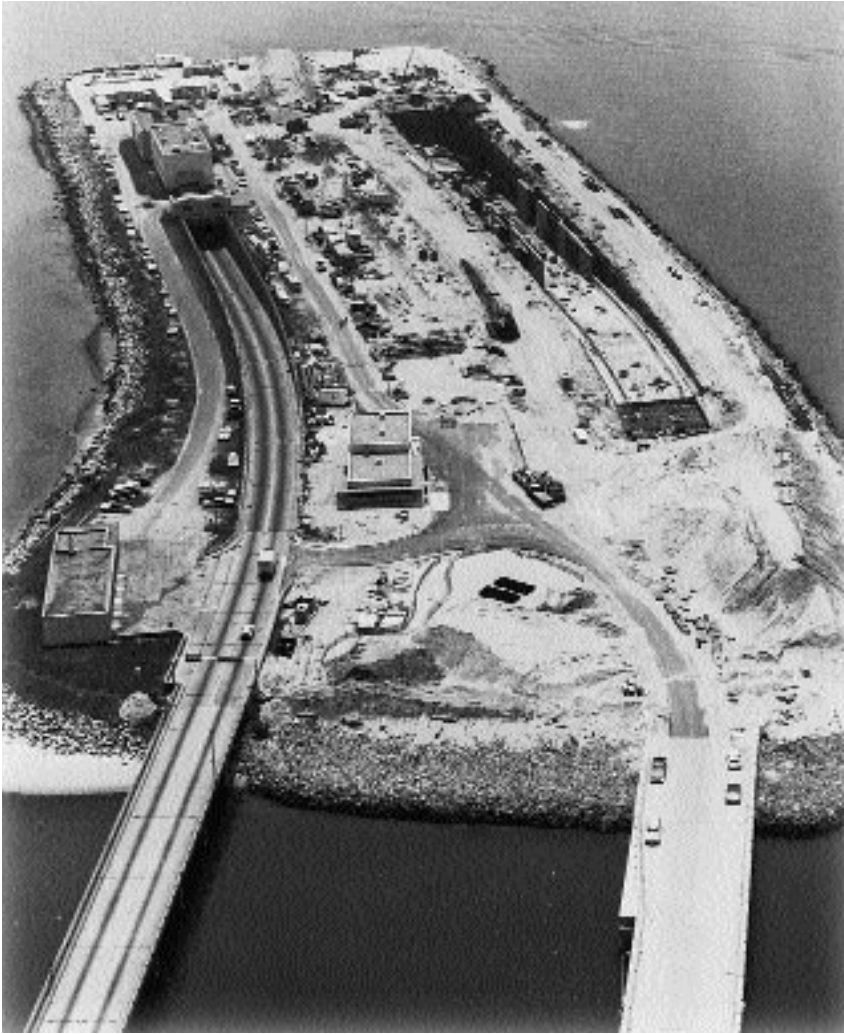
The second Hampton Roads Bridge-Tunnel was under construction in 1973.
