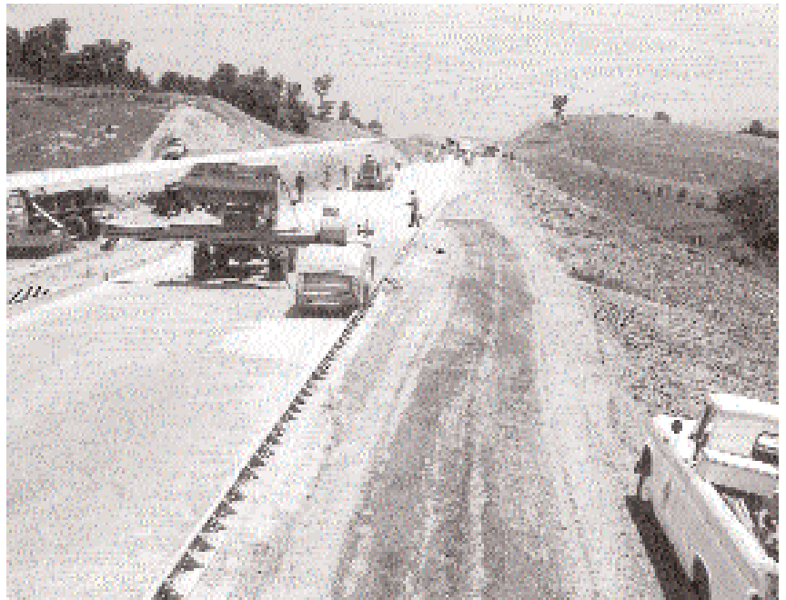
Interstate construction progresses along the I-81 corridor.
