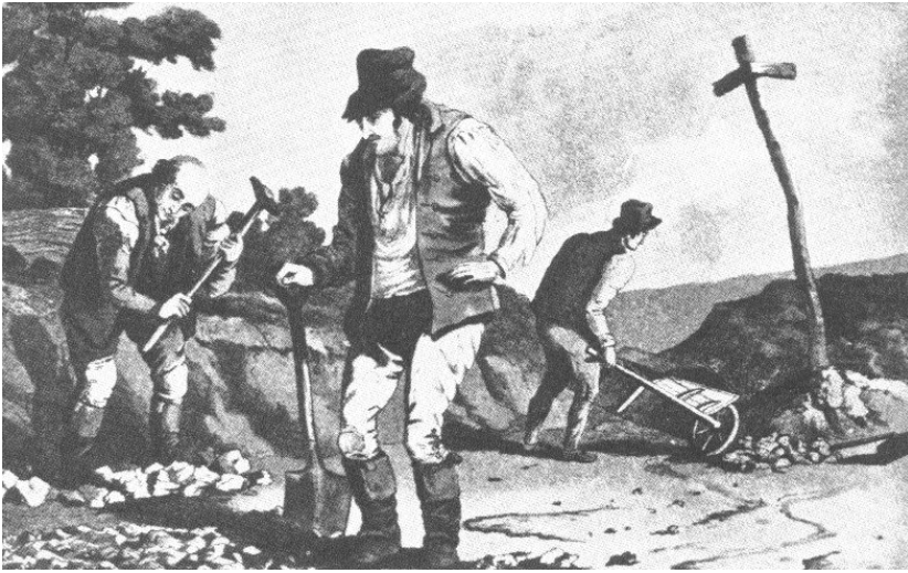
Much manual labor was the requirement for building and maintaining early roads.
