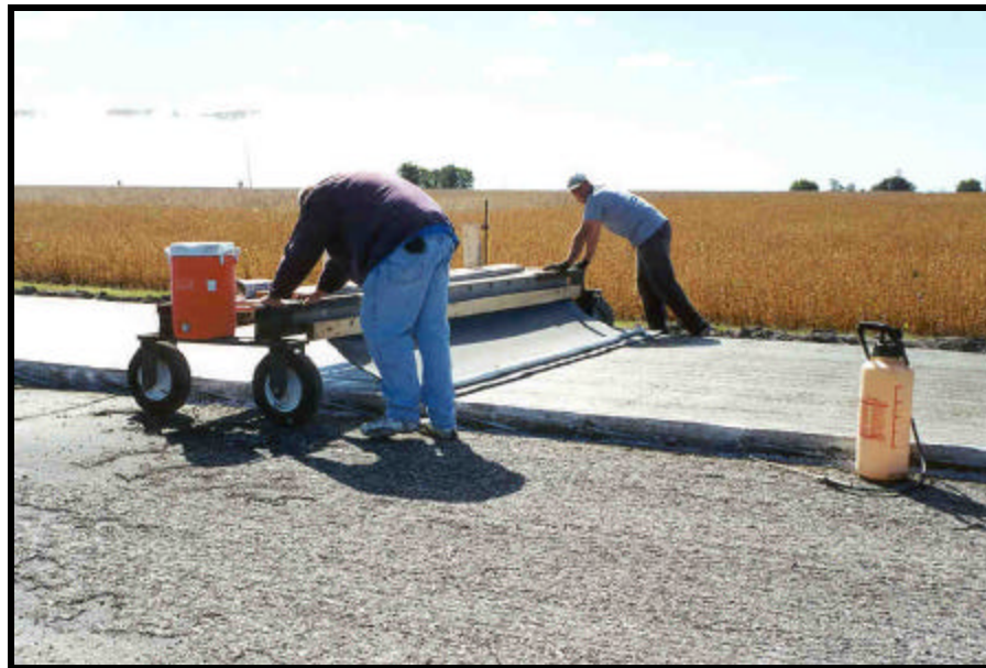
Figure 26. Longitudinal Astroturf Drag
