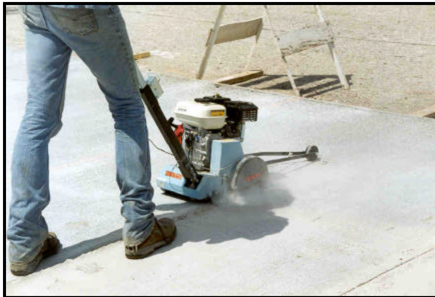
Figure 15. Early Entry Saw Used For Partial-Depth Cuts
