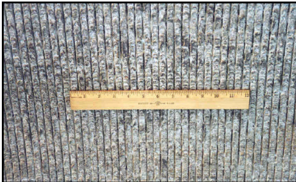
Figure 28. Transverse Tine Spacing
