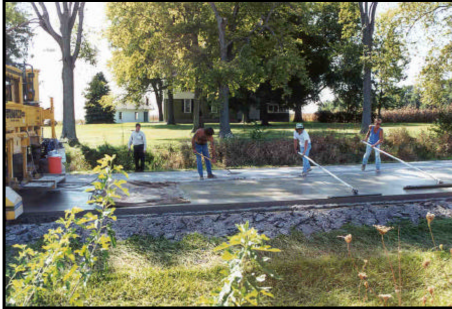
Figure 25. Concrete Finishing Techniques
