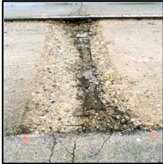
Figure 10. Partial-Depth Patch
