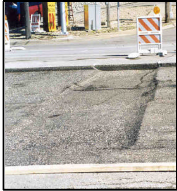
Figure 4. Partial-Depth Patch
