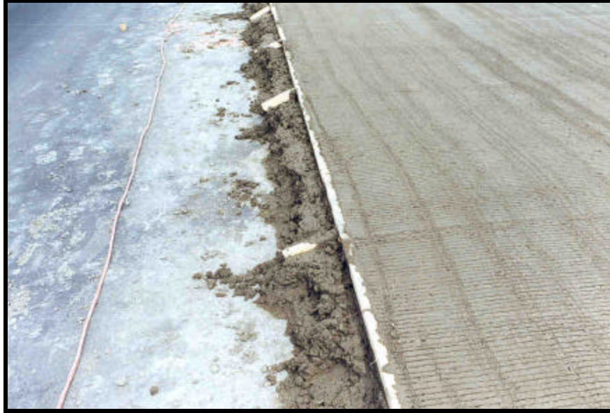
Figure 22. Concrete Flow Under Form Work
