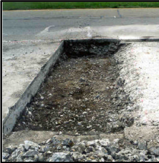
Figure 9. Full-Depth Patch
