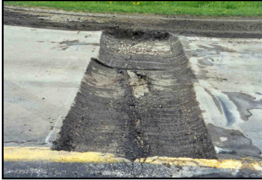
Figure 19. Milled Out Area For Bituminous Patch
