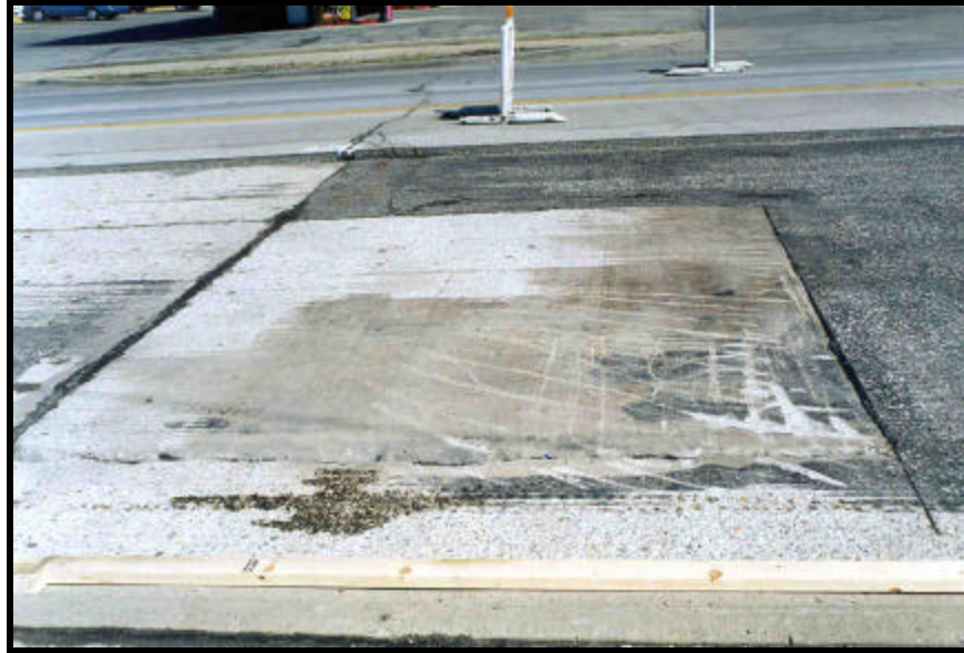
Figure 2. Bituminous To Concrete Pavement Transition
