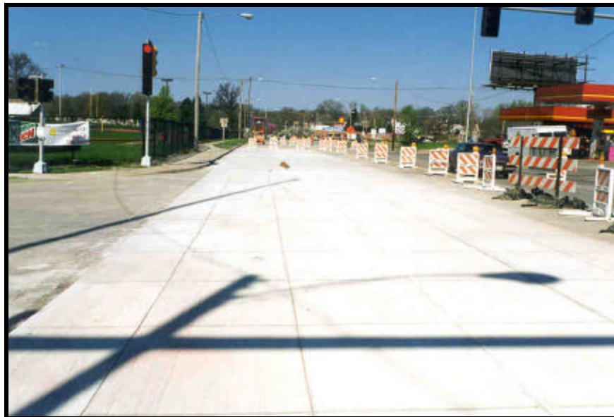
Figure 6. Completed Partial-Depth Saw Cuts
