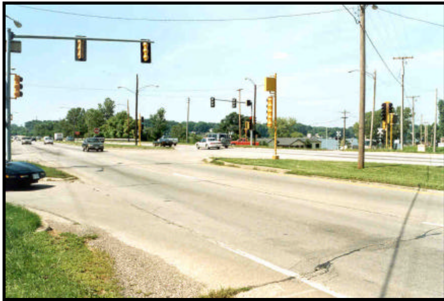
Figure 7. U.S. Highway 36 And Country Club Road (Looking West)
