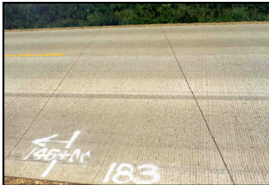
Figure 24. Partial-Depth Saw Cut Pattern
