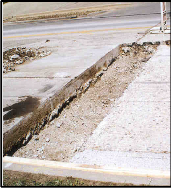
Figure 3. Full-Depth Patch
