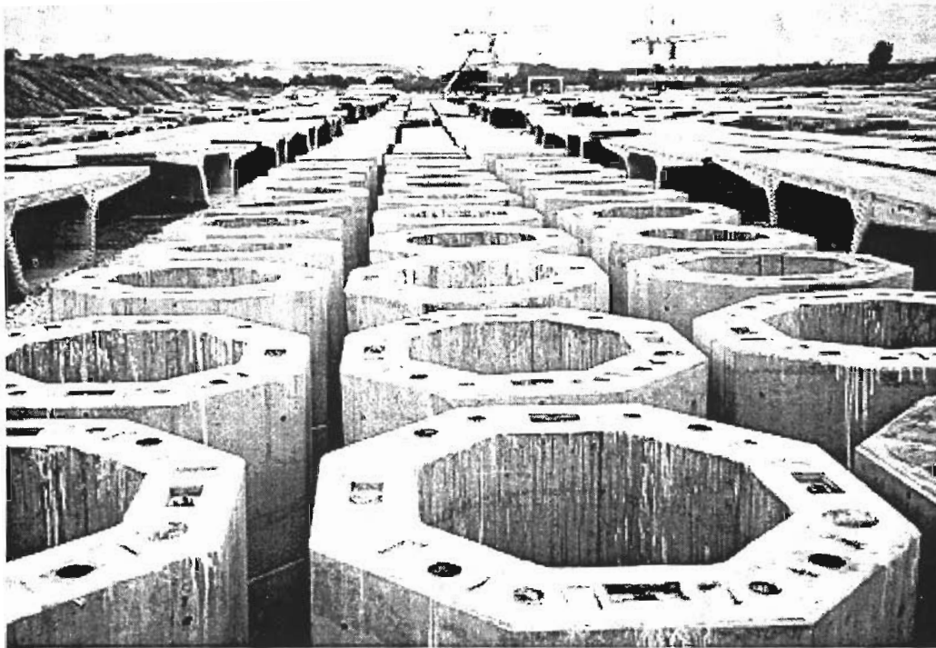
Figure 4.6 Completed pier segments in storage at the casting yard.
