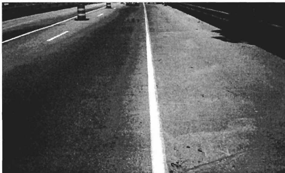
Figure 2.3. Bridge 2 prior to overlay placement. The modified EP5 epoxy overlay is in excellent condition.
