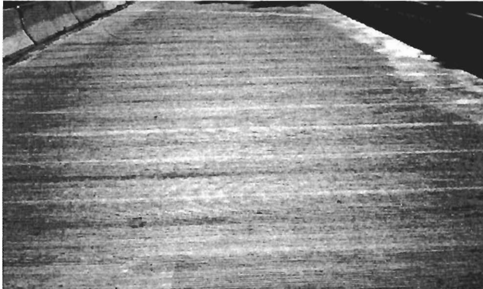
Figure 5.7. Outside lane and shoulder of Bridge 5 after ML overlay placement.
