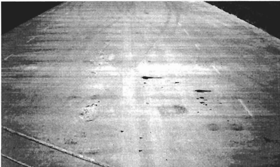
Figure 5.8. Outside lane and shoulder of Bridge 6 after LMC overlay placement.
