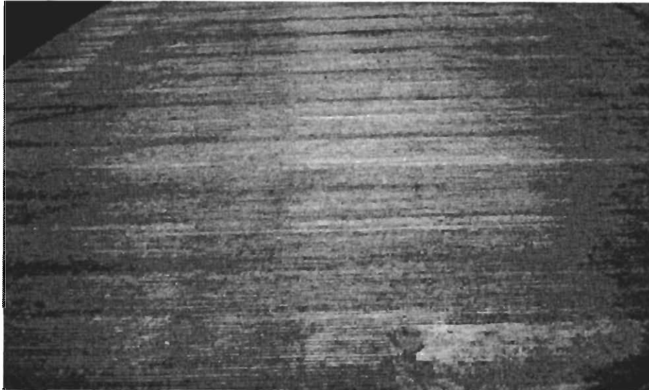
Figure 5.3. Outside lane and shoulder of Bridge 1 after SF overlay placement.
