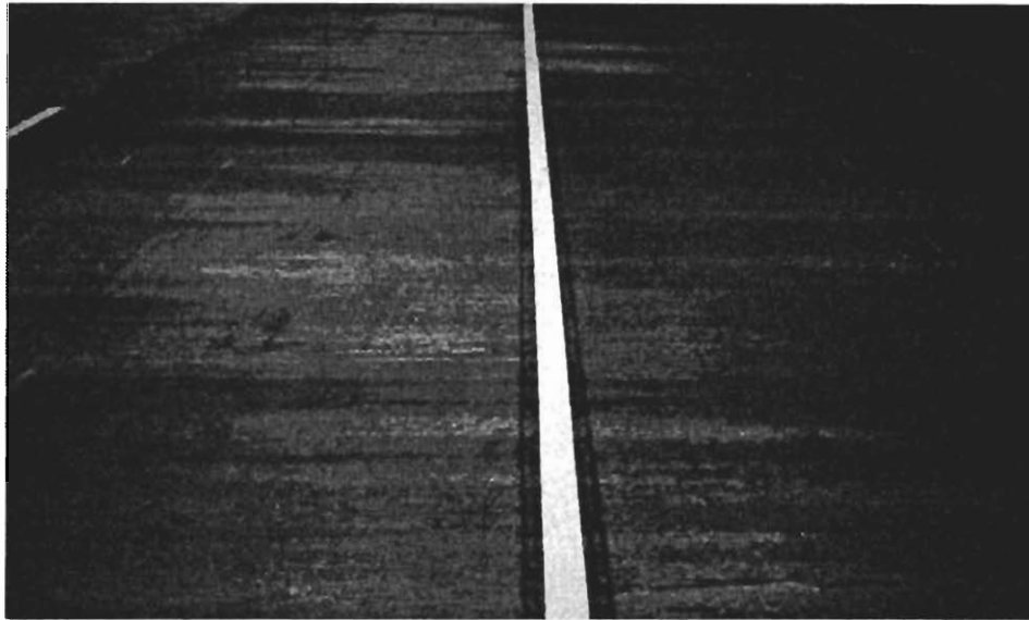
Figure 5.5. Outside lane and shoulder of Bridge 3 after LMCHE overlay placement.
