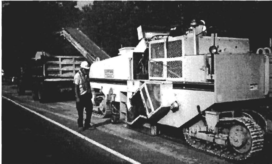
Figure 3.1. Milling machine removing the top 13 mm (0.5 in) of Bridge 4.
