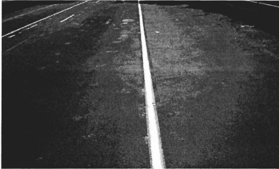
Figure 2.4. Bridge 3 prior to overlay placement.
