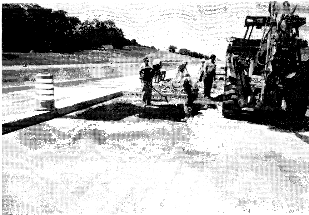
Figure 33. Replacing disturbed subbase with asphaltic concrete.
