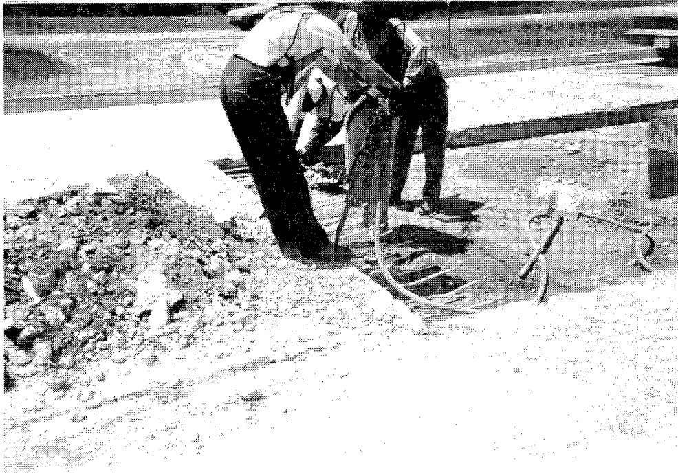
Figure 29. End section removal – using a jackhammer.
