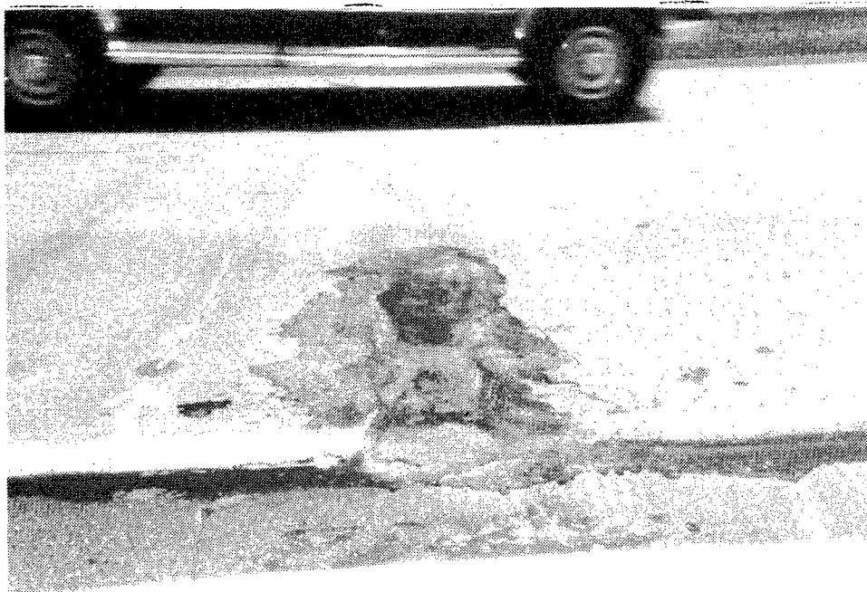
Figure 21. Punchout marked out for removal.
