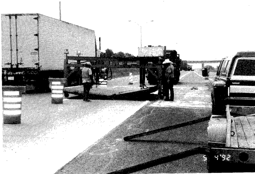
Figure 27. Slab lifting device.
