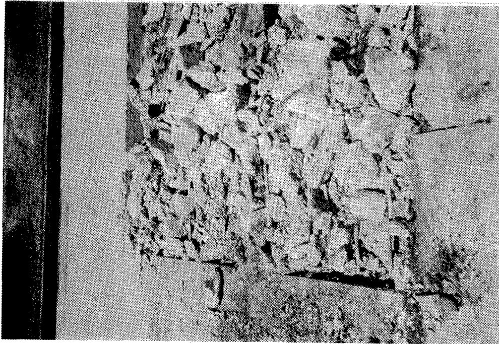
Figure 31. End section removal - close-up view.
