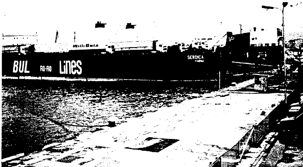
Photo 3-11 Port of Varna, Ro-Ro Berth
