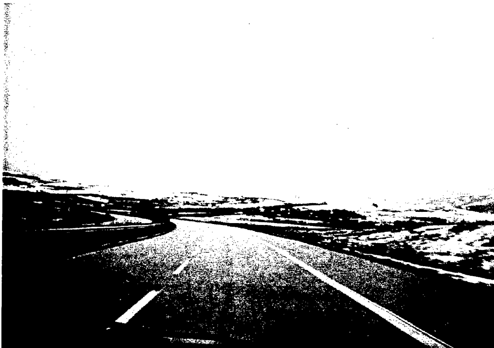
Photo 3-7 Segment of Route E-772, Sofia – Varna; A4 Lane Divided with Good Geometrics
