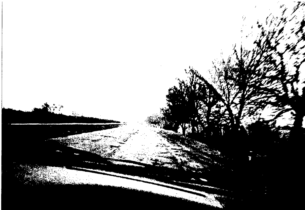
Photo 3-5 Section of Route E-773, Burgas - Stara Zagora
