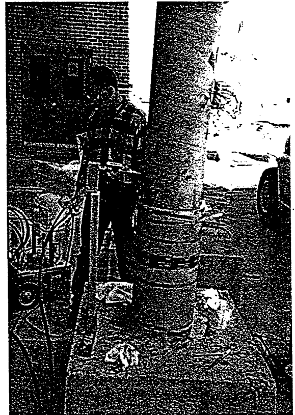
c) Pressurizing the Gap Between the FRP Composite and Concrete Surface with Epoxy Resin
