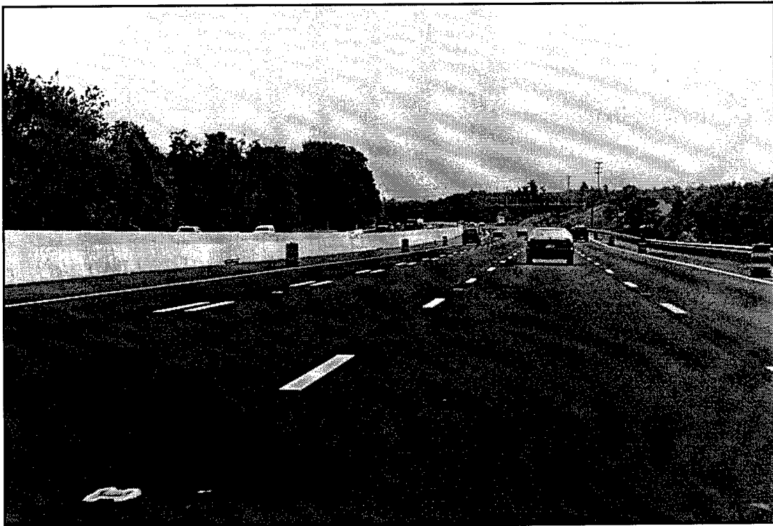
Figure 17. Pavement Marking for Concurrent HOV Lane on I-66
