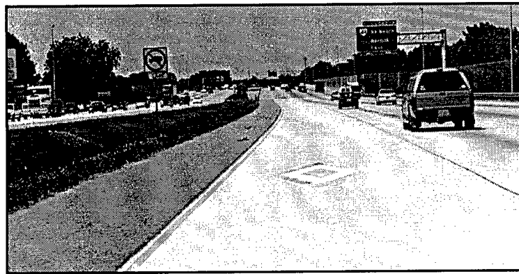
Figure 21. Pavement Marking for Concurrent HOV lane, I-64
