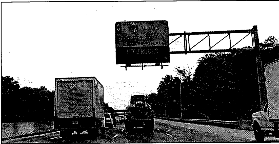
Figure 16. Variable Message Sign, I-66 Inside the Beltway
