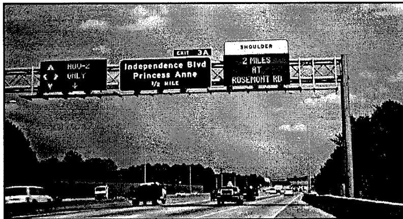
Figure 27. VMS Message No. 2 for Shoulder Lane Use, Rt. 44
