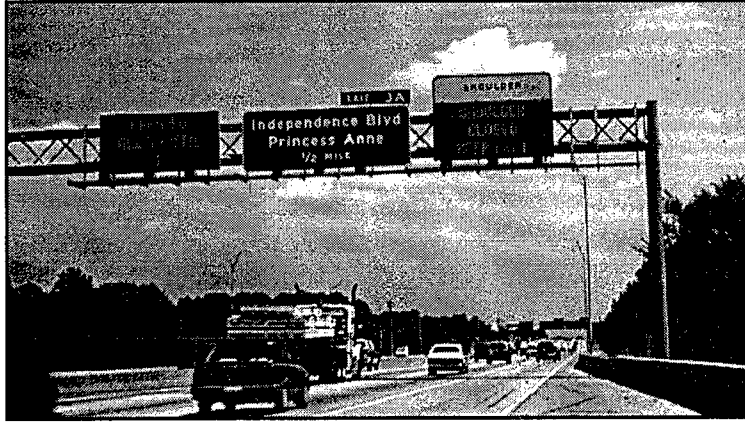
Figure 25. Variable Message Sign for Shoulder Lane Use, Rt. 44
