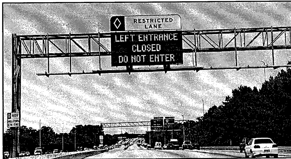
Figure 22. Variable Message Signs used for HOV Information
