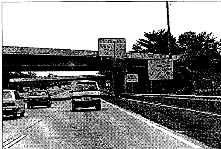
Figure 9. Lane Control Signal with Static Informational Sign
