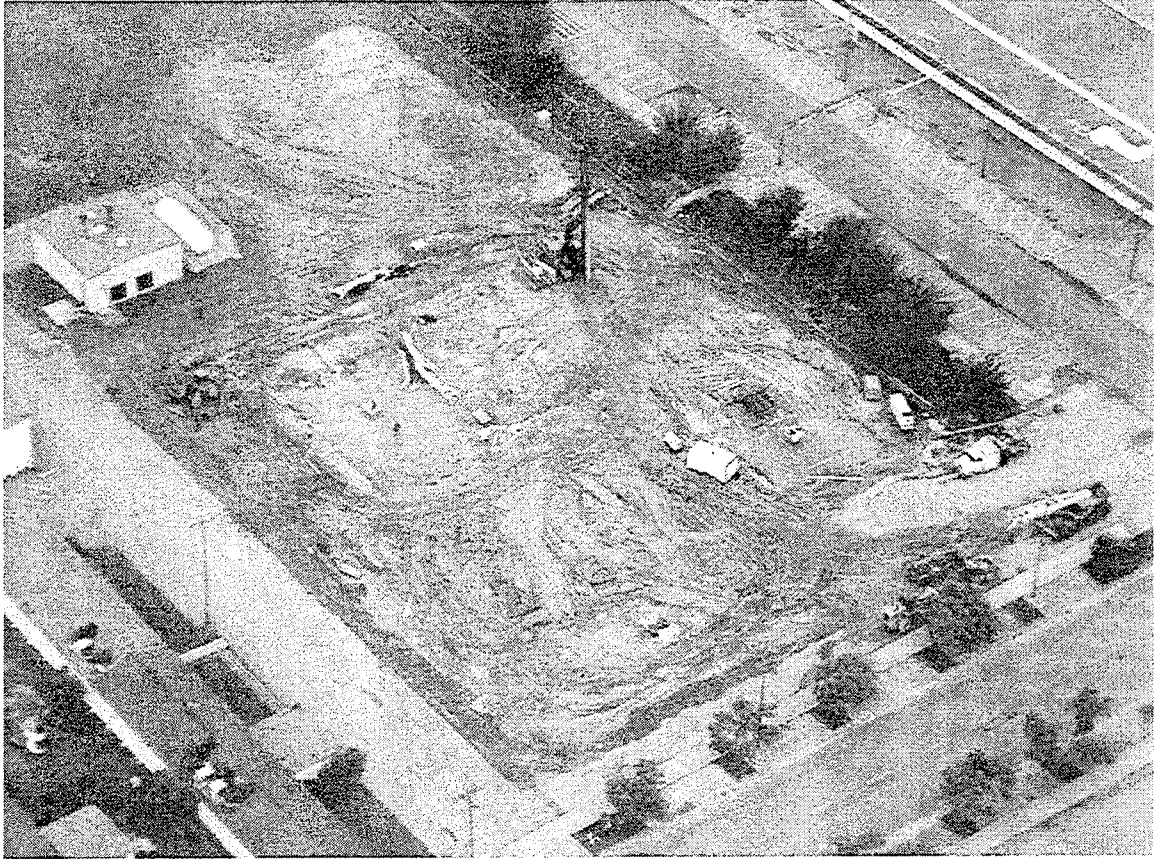
Figure 1.2 Aerial Photograph of Treasure Island Liquefaction Test Site
