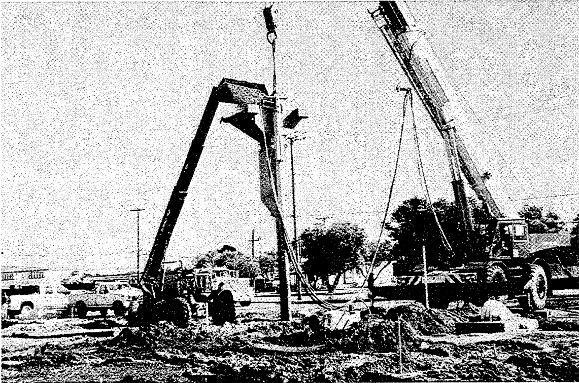
Figure 4.32 Installation of Stone Columns
