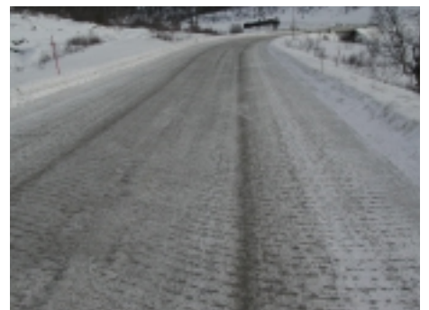
Figure 3. Typical pattern on the road when using warm wetted sand and a spinner.
