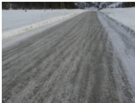
Figure 2. Typical pattern on the road when using warm wetted sand and a roller distributor.
