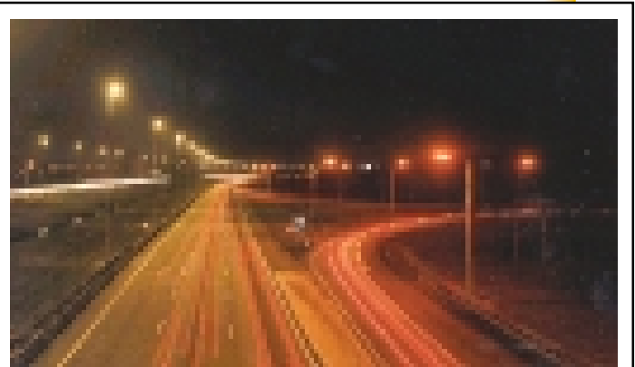
Figure 56. Normal level of roadway lighting.
