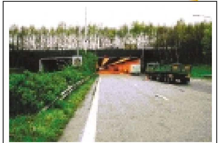
Figure 17. Wevelgem Tunnel, Belgium.
