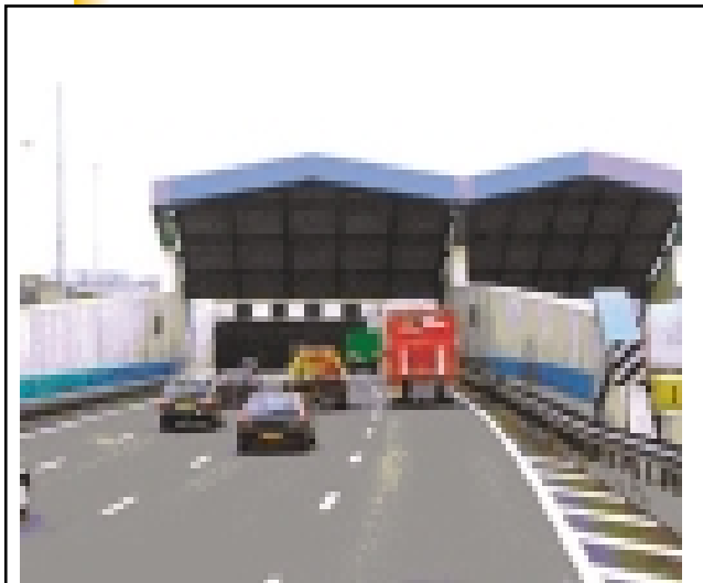
Figure 28. Tunnel at Schiphol Airport, the Netherlands. The sunscreens are not actually needed, because of the counter-beam threshold lighting. They were left in place for aesthetic reasons.
