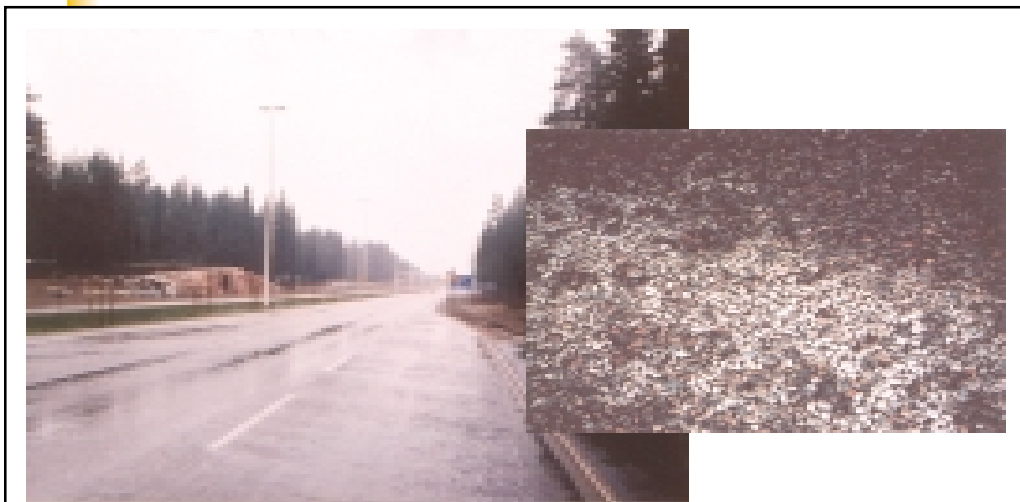
Figure 23. Wet roadway in Finland (inset, close-up of pavement).
