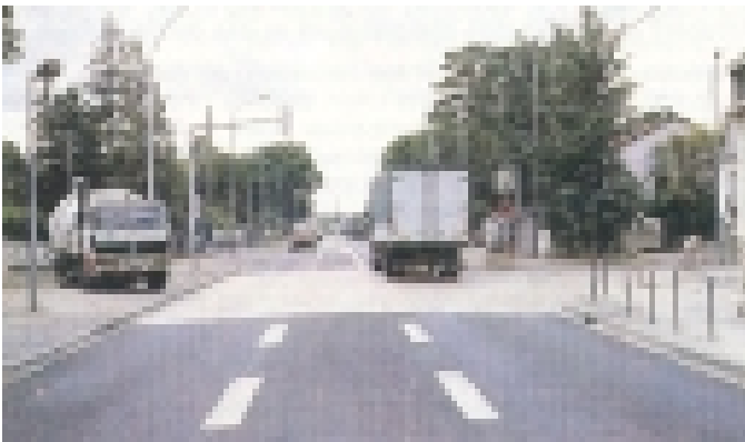
Figure 61. & 62 Application of colored pavement.
