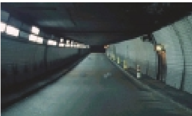
Figure 63. Typical motorist's view of tunnel.
