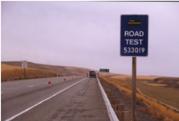
Figure 3.1.16 Overview of test site 53-3019.
