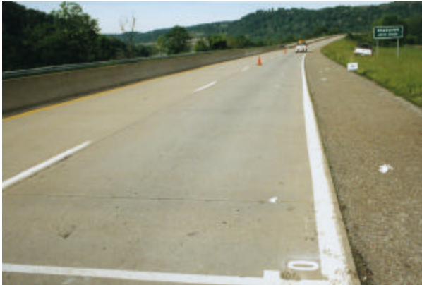
Figure 3.1.24 Overview of test site 39-3801.
