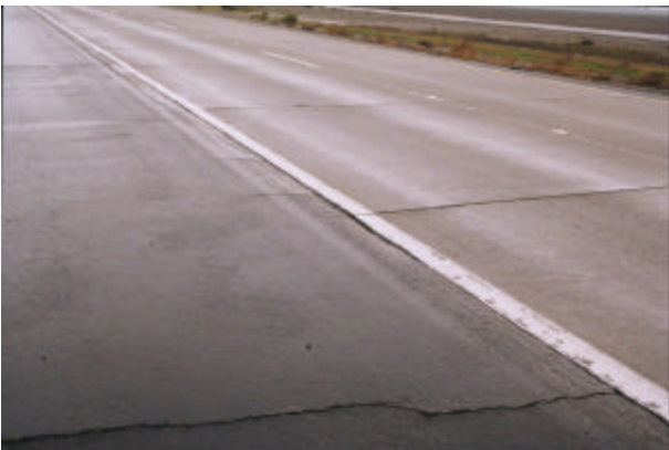
Figure 3.1.9 No slab distress at test site 06-7456, Tracy Test Road.
