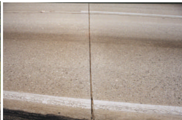
Figure 3.1.33 Distress free transverse joint at 13-GA1-5.
