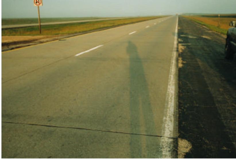
Figure 4.3.13 Overview of test section 19-3055.
