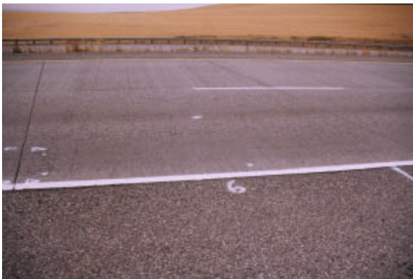
Figure 3.1.17 Typical distress free slab at 53-3019.
