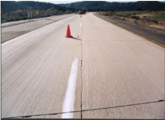
Figure 3.1.7 Distress free slab at test site 06-3021.
