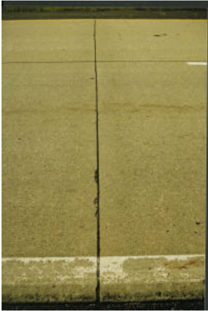
Figure 3.1.21 Transverse joint in good condition at 19-3055.
