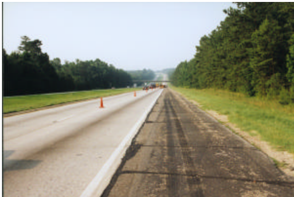
Figure 3.1.32 Overview of test site 13-GA1-5.
