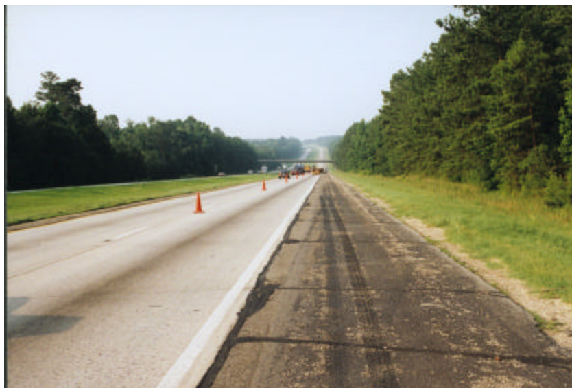
Figure 4.3.10 Overview of the Georgia test section, 13-GA 1-5.
