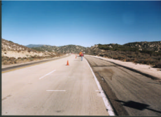
Figure 3.1.6 Overview of test site 06-3021.
