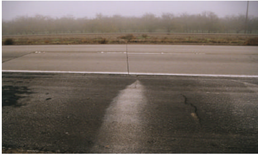
Figure 4.2.3 Surface staining on the shoulder close to joints from Tracy Test Road (06-CS1).
