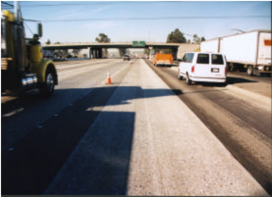
Figure 3.1.14 Overview of test site 06-I-10.
