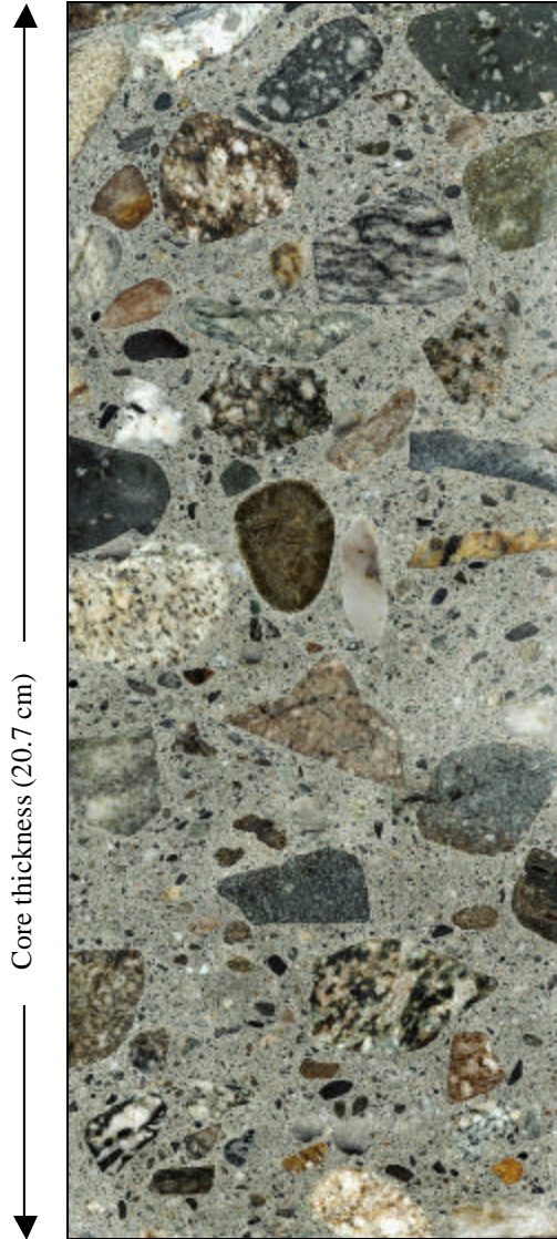
Figure 3.2.6 Polished cross-section of pavement section 06 I-10.
