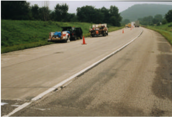
Figure 3.1.22 Overview of test site 27-4054.
