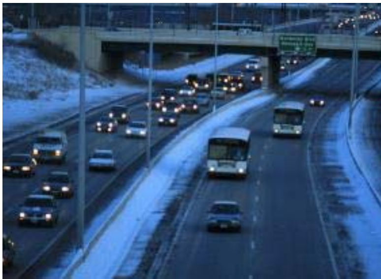
Figure 2. Reversible HOV Flow Lane in the Center of I-394 in Minneapolis (10).
