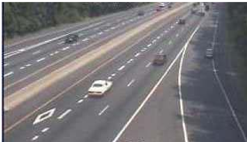
Figure 4. Concurrent HOV Lane Along I-270 in Maryland ( 14 ).
