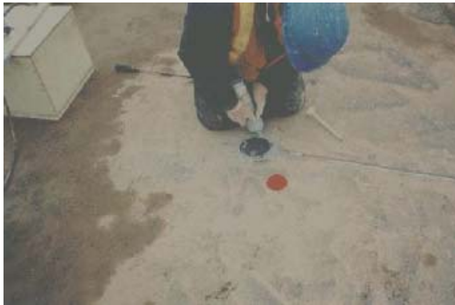
Figure 2. Installation of an SSI Pavement Sensor
