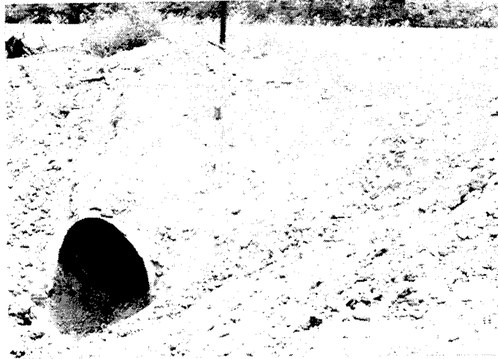
Figure 14 The buried culvert with the test station in place.
