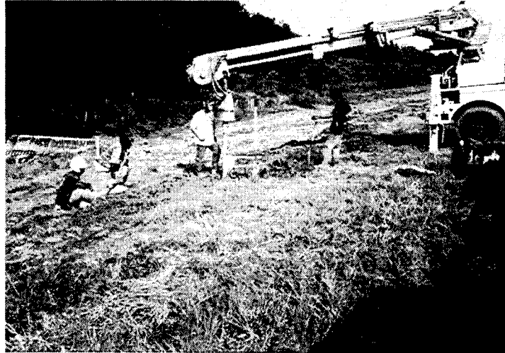
Figure 6 Hole being drilled for installation of two external anodes
