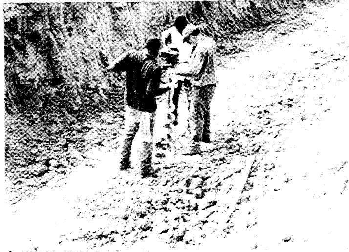
Figure 10 Manual digging of holes for installation of external anodes.
