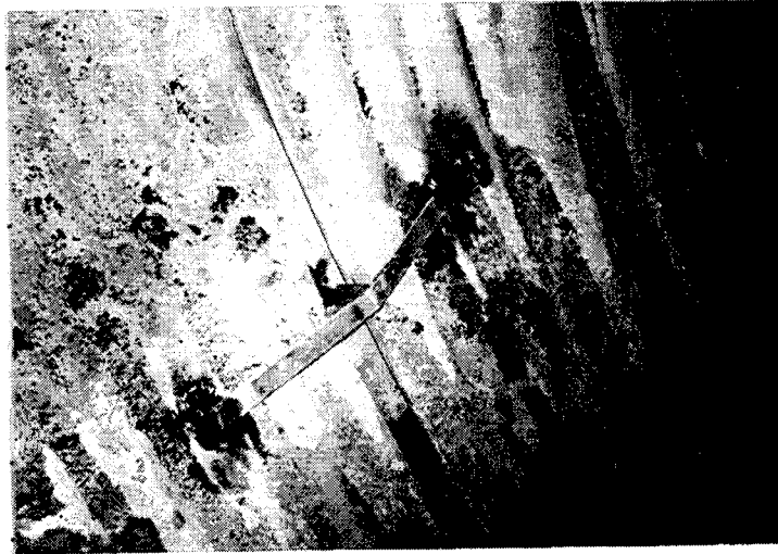
Figure 4 Metal strap used to electrically connect the culverts and band
