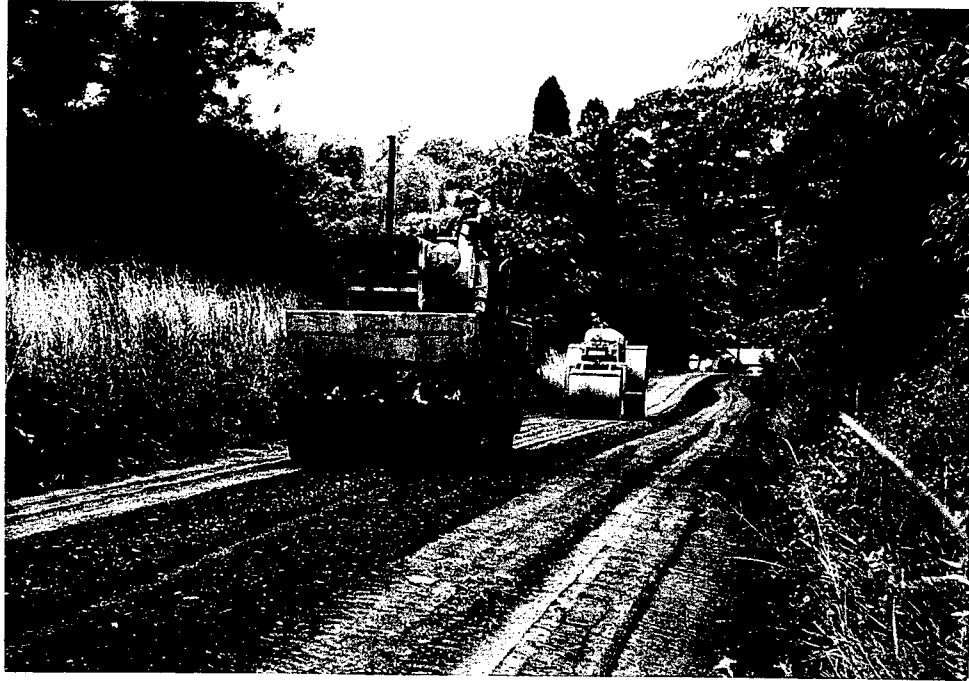
Photo 11 – Construction Photo taken July 1992.
