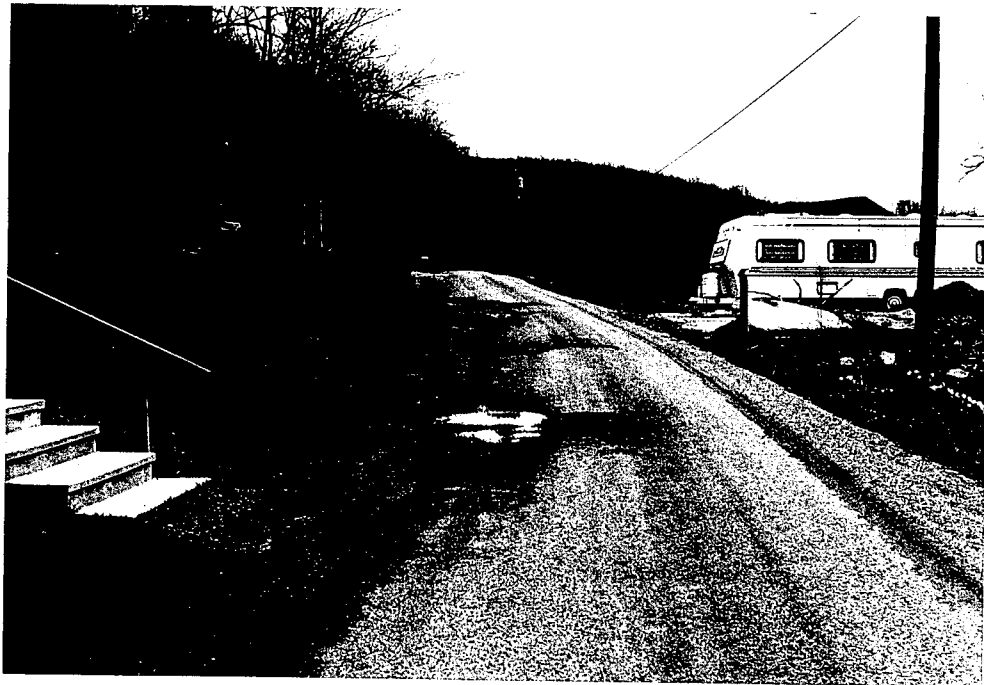
Photo 8 – Inspection Photo taken April 1994 showing potholes.
