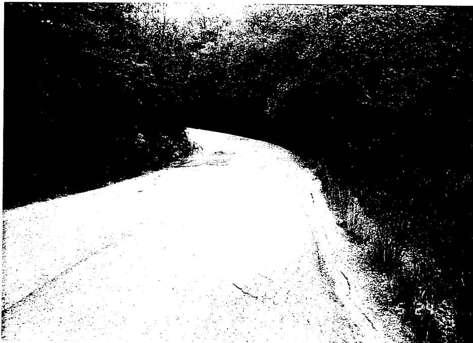
Photo 16 – Inspection Photo taken May 1995.
