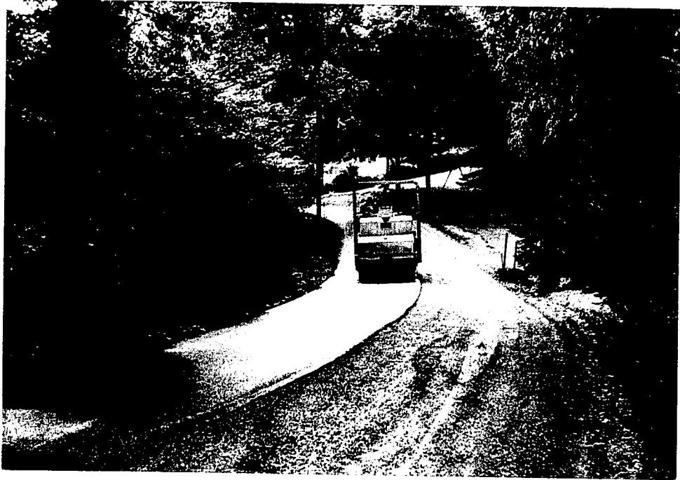
Photo 35 – Construction Photo taken September 1992.
