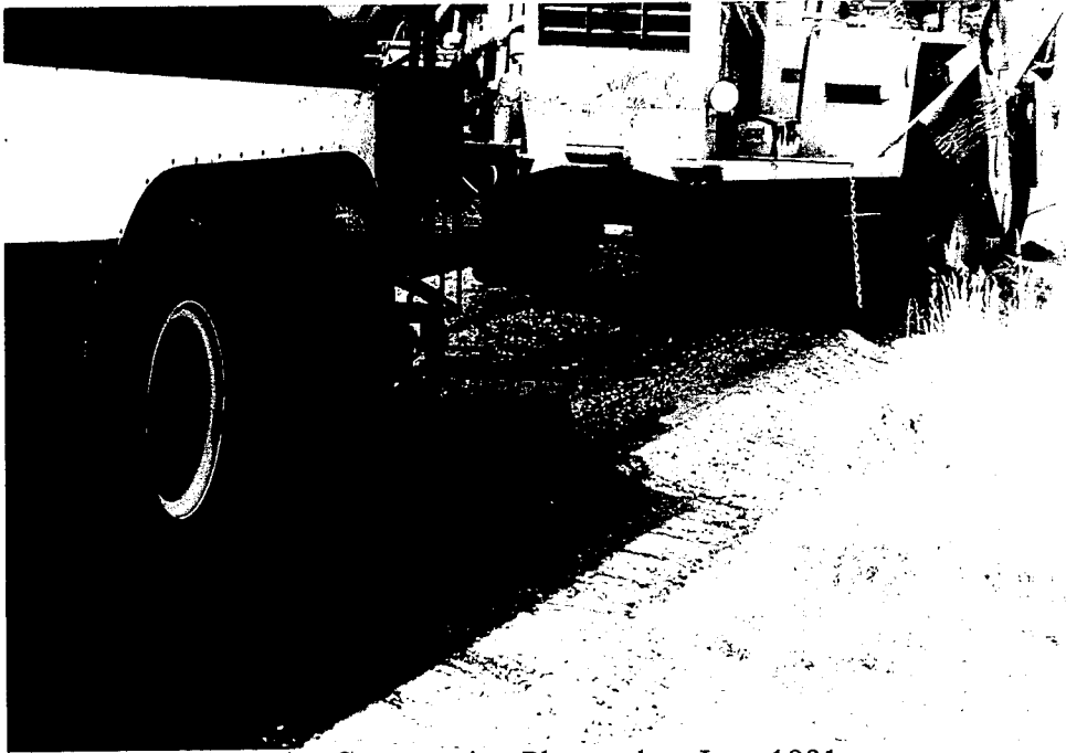
Photo 1 – Construction Photo taken June 1991.
