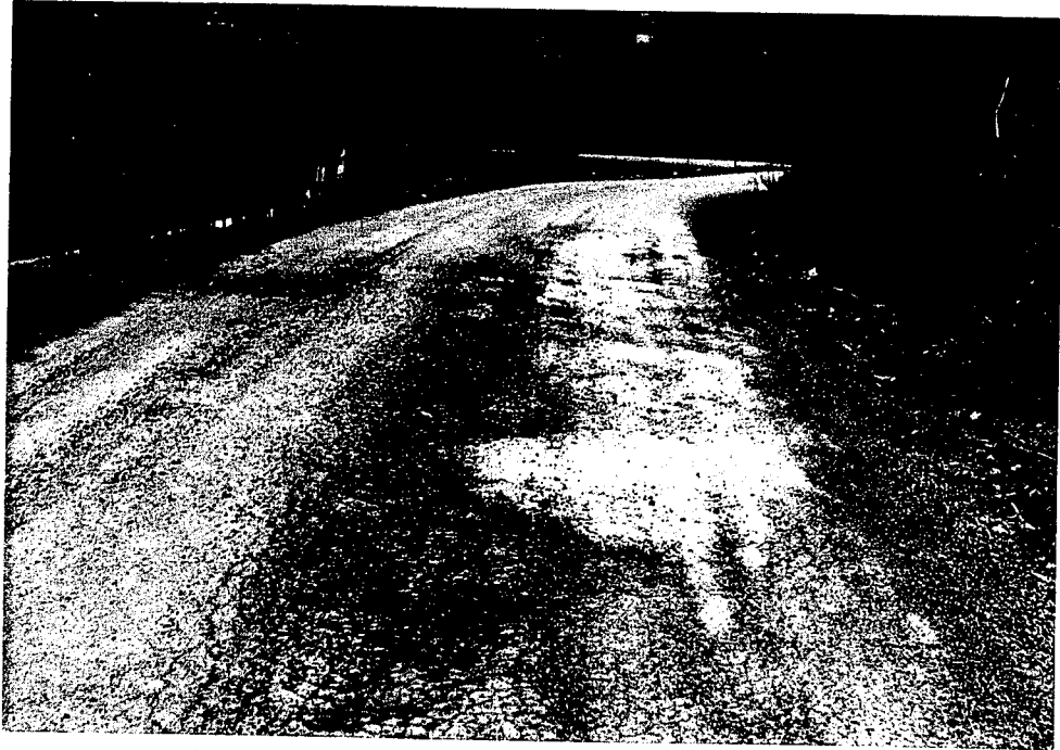
Photo 3 – Inspection Photo taken March 1993.
