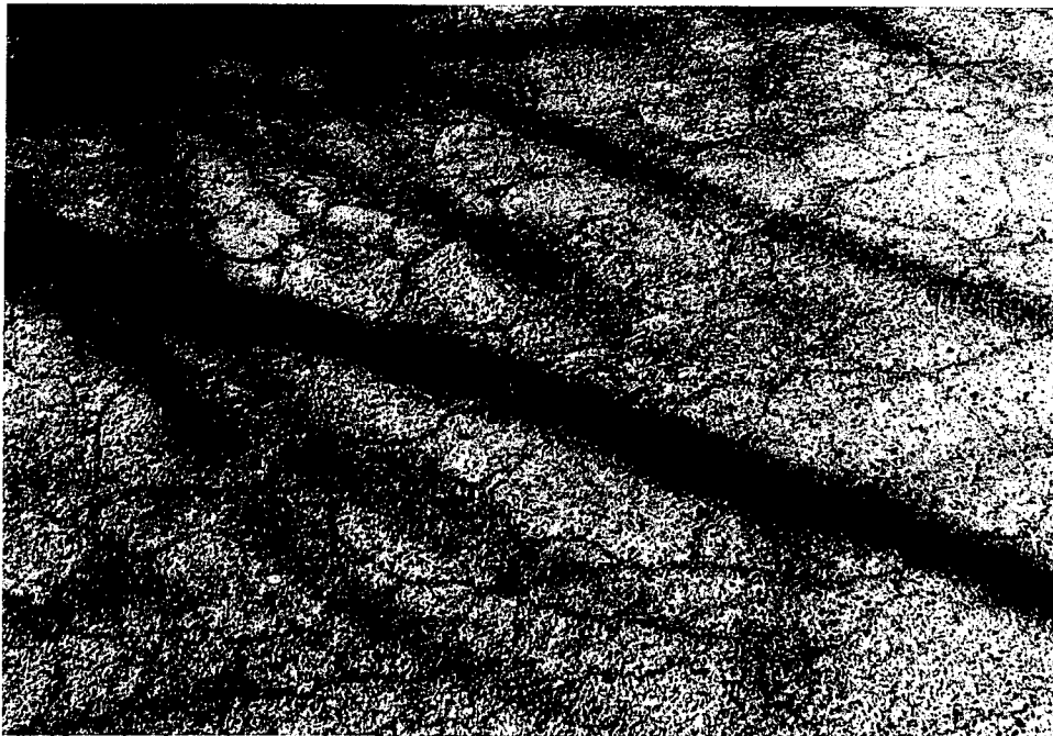
Photo 14 – Inspection Photo taken April 1993 showing alligator cracking.
