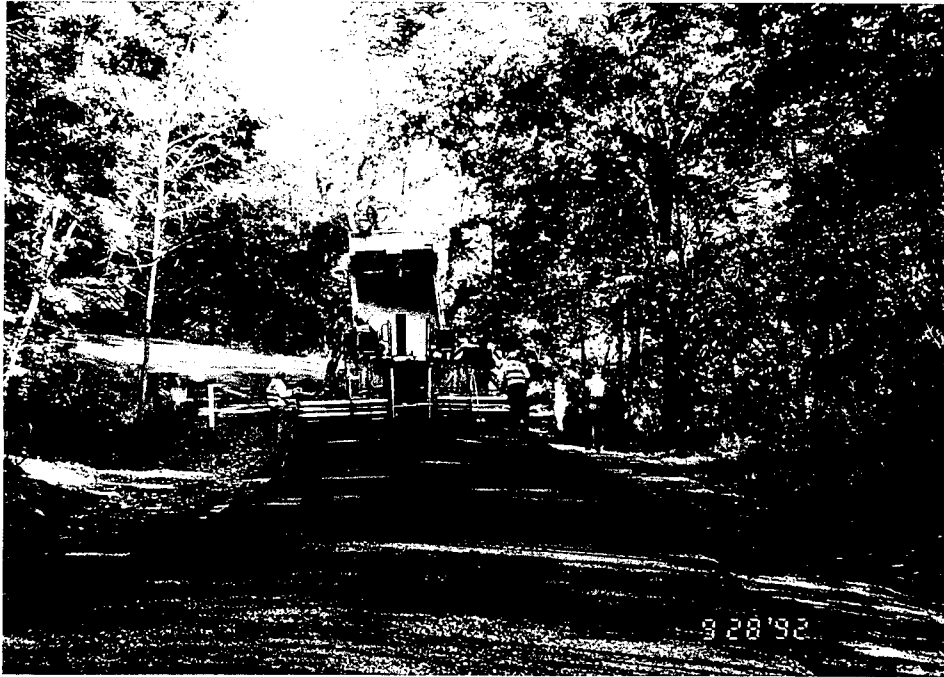
Photo 17 – Construction Photo taken September 1992.
