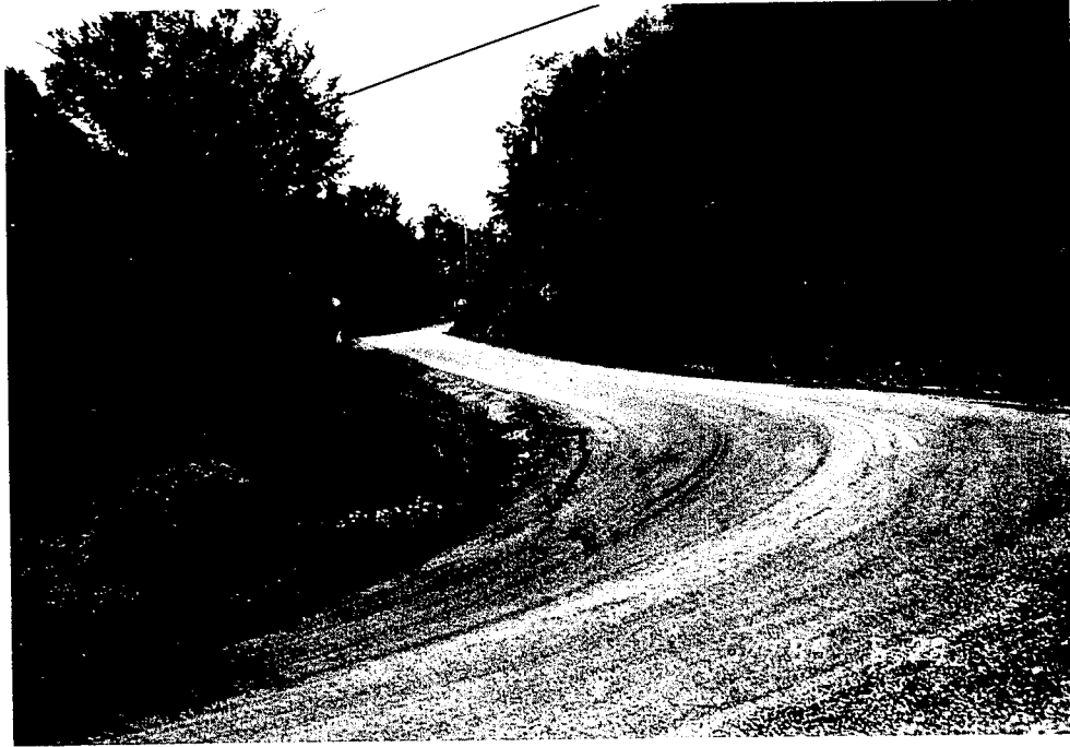
Photo 23 – Inspection Photo taken April 1993.
