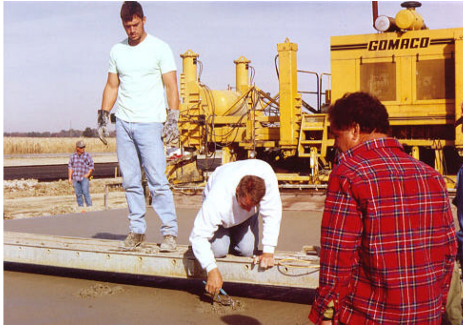
Figure 12.14 Pulling Protective Boxes
