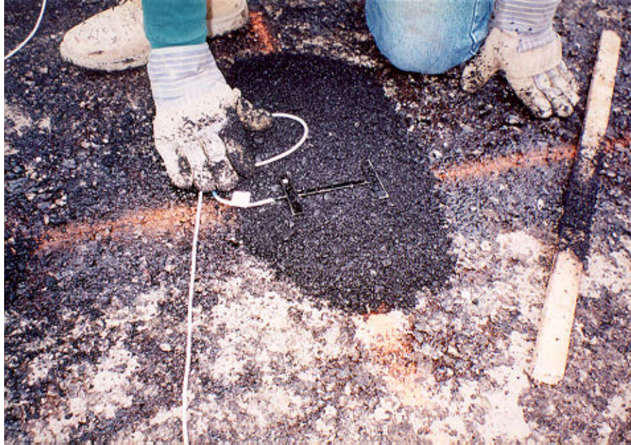
Figure 12.16 Sensor Placement in AC Pavement Sections
