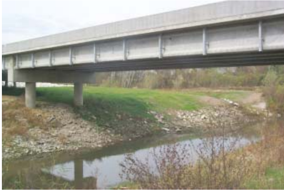
Figure 10.b. Photograph of Bridge #2.
