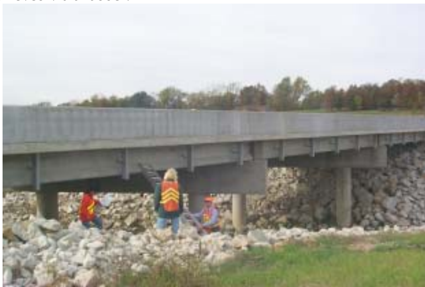
Figure 14. Ladders provided access to the sensor housings.
