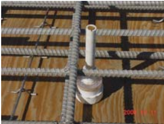
Figure 2. Sensor Housing Attached to Forms of CIP Deck
