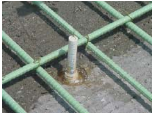
Figure 3. Sensor Housing Glued into Deck Panel Core Hole
