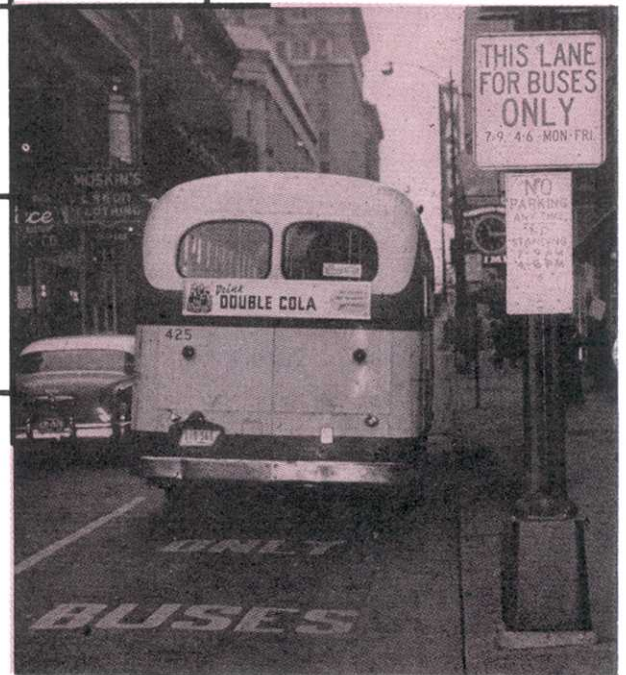
Bus lane with appropriate signs.
