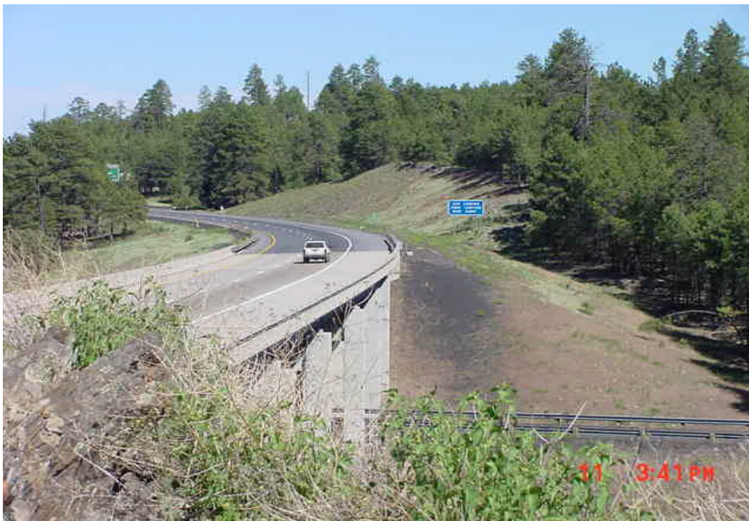
Figure 5. A View of Riordan Bridge Looking East from the RWIS site.
