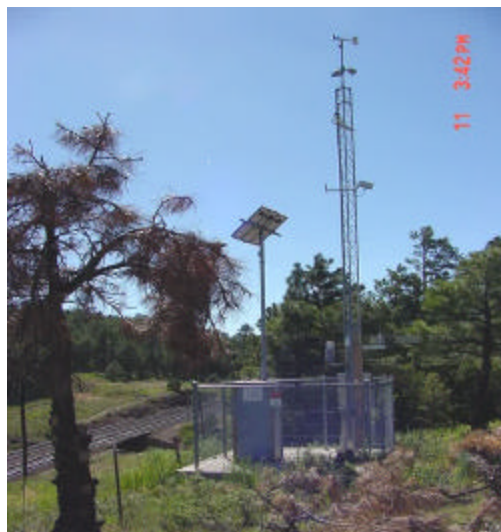
Figure 1. The Riordan RWIS Test Site
