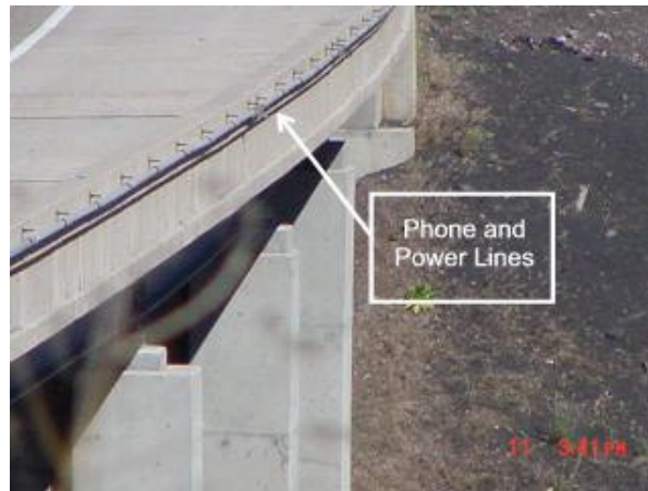
Figure 3: New Telephone and Power Lines Installed on Riordan Bridge
