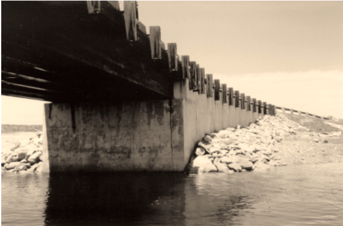
Figure 1—Creosote loss from treated glulam beams used in constructing a highway bridge across Narragansett Bay.
