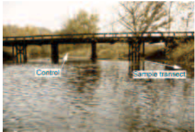
Figure 13—Bridge 148 over Pipe Creek viewed from downstream.
