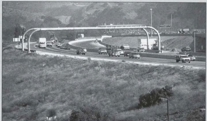
'Overhead gantries electronically record usage so there is no stopping at toll booths'
