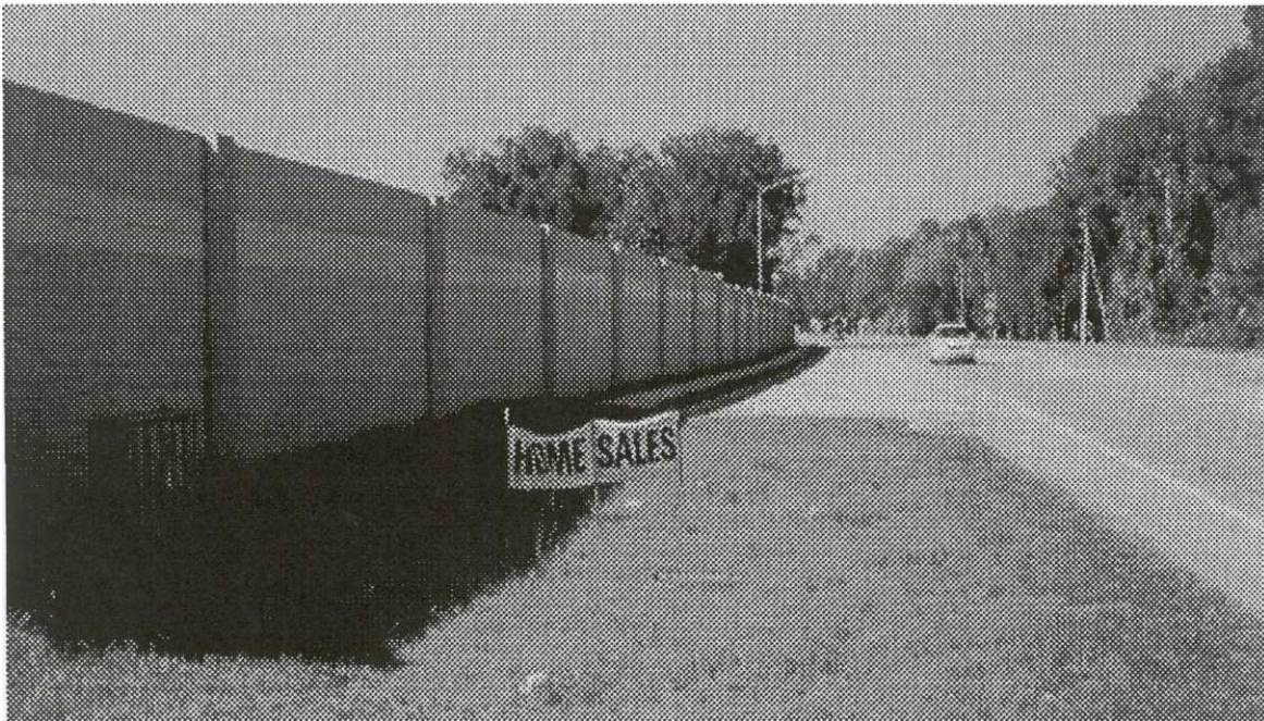
Roadway View of Noise Wall
