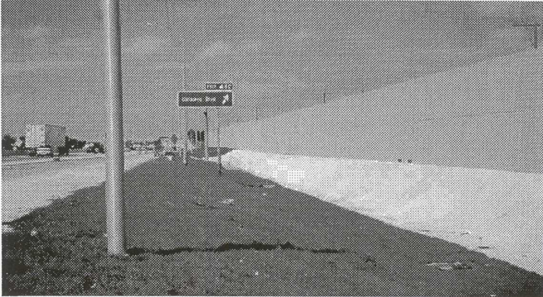
Roadway View of Noise Wall
