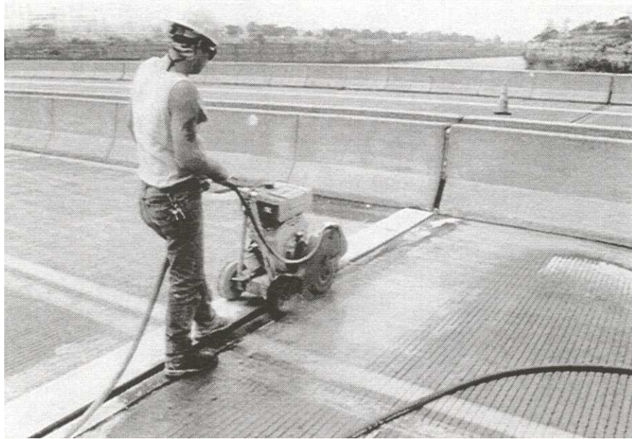
Sawcutting adjacent to the joint.
