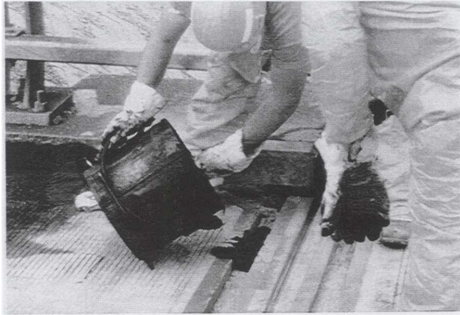
Placing the elastomeric concrete header material.
