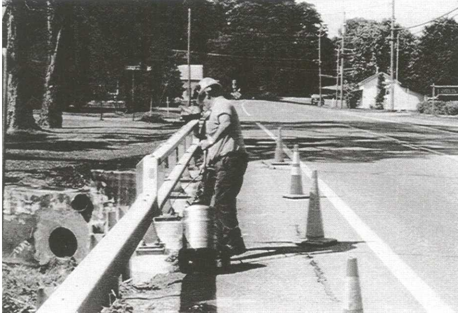
Typical equipment (portable spray unit).
