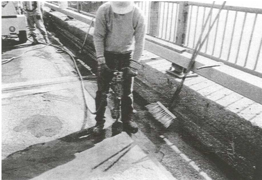
Remove existing asphalt wearing surface.
