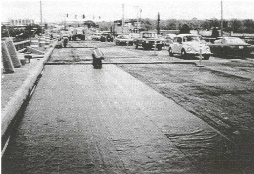
Place waterproof membrane.
