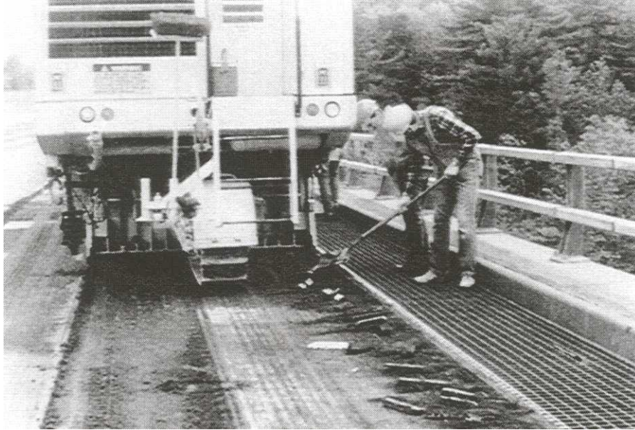
Remove existing wearing surface
