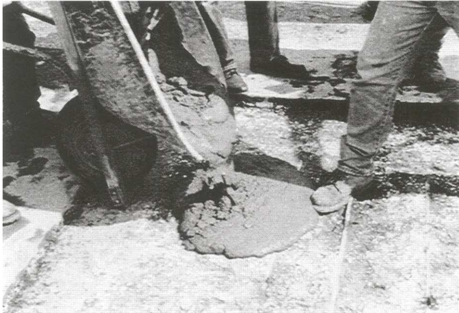
Placing repair material.
