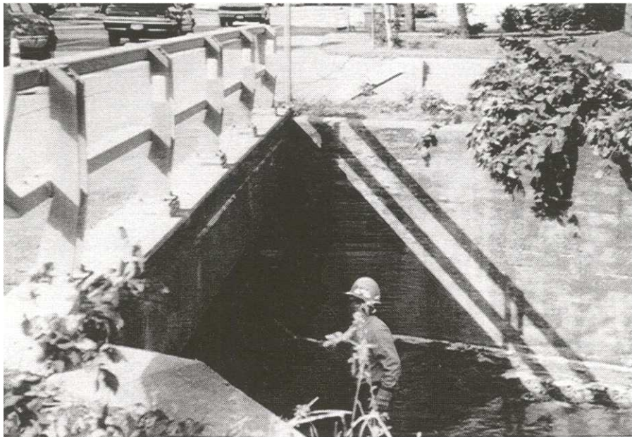
Applying penetrating sealer.
