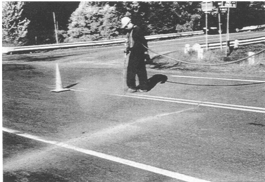
Clean out crack with compressed air.
