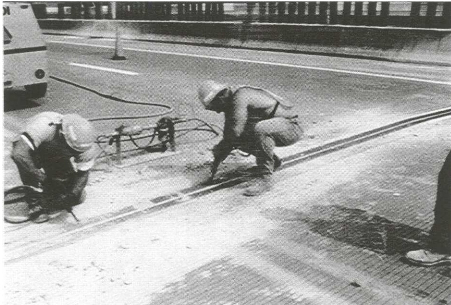
Removing concrete adjacent to the joint.
