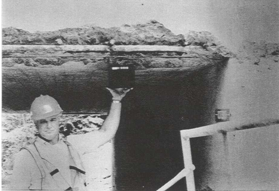
Determine extent of deteriorated concrete.
