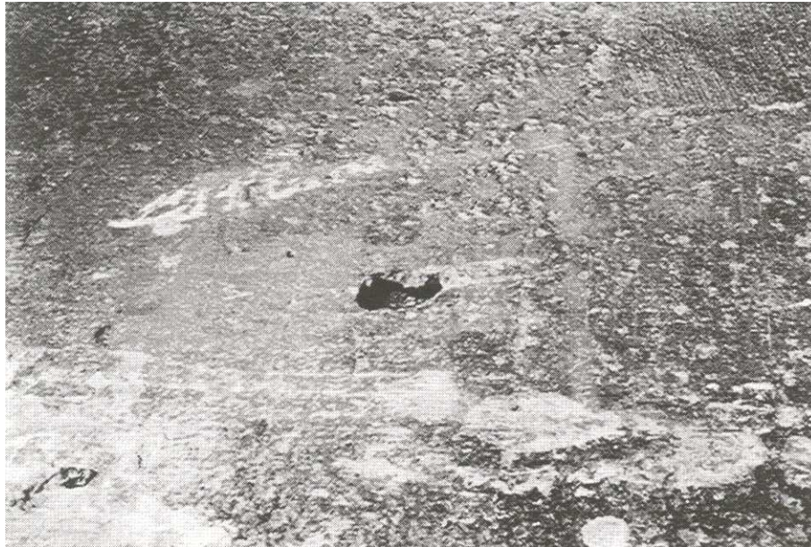
Marking edges of proposed patch.
