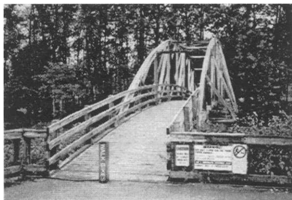
Pedestrian Bridge Over Sammamish River
