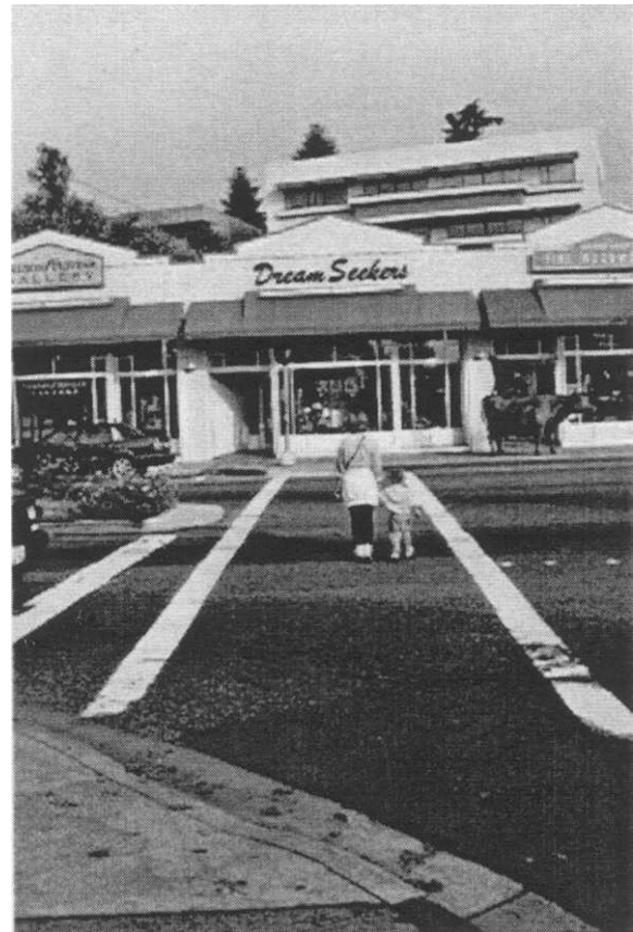
Typical Marked Crosswalk at Intersection
