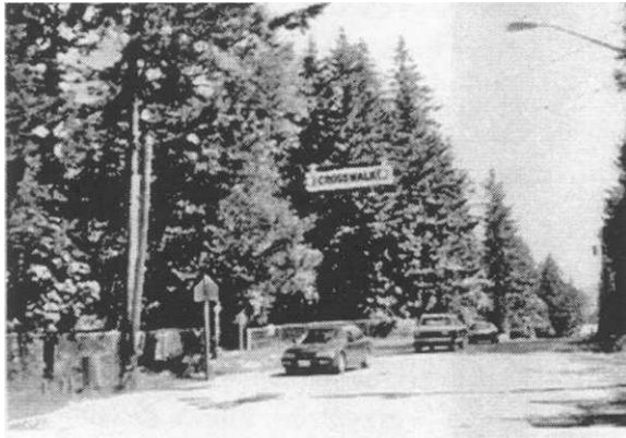
Overhead Flashing Beacon
