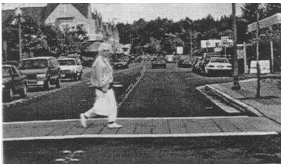
Raised Mid-Block Crossing
