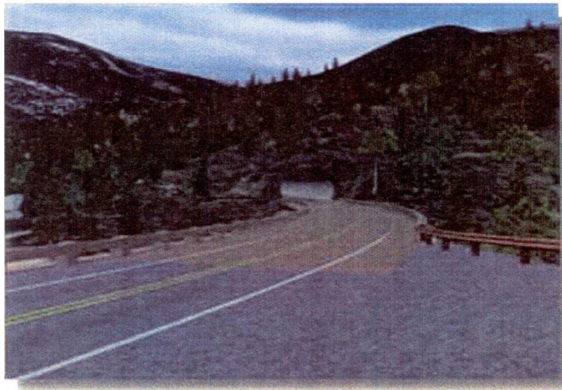
Figure 38. Tunnel Alternative From Guanella Pass Project as Displayed on Project Web Page.
