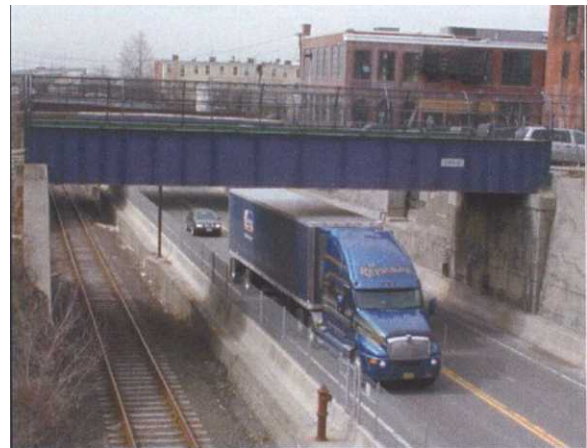
Figure B.01. The Boston Haul Road was created from an underutilized railroad alignment.
