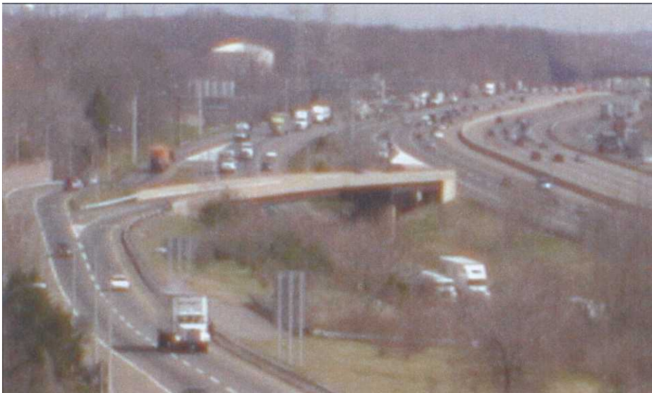
Figure 3.05. The New Jersey Turnpike. Photo shows the outer roadways carrying trucks, while most automobiles use the inner highway. The flyover (center-left) connects the inner highway to the exit ramp.
