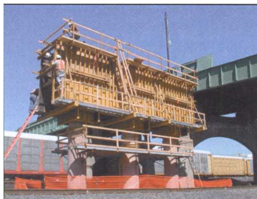
Figure 3.07. Doremus Ave. bridge reconstruction.
