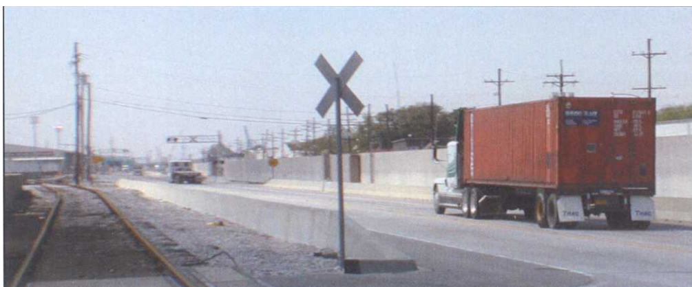
Figure 3.02. The Tchoupitoulas Roadway, Port NOLA. Photos show the flood wall and realigned railroad.
