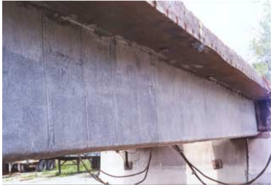
(a) Overall View
