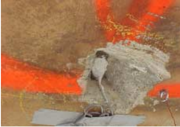
(a) Strain Gage on Reinforcing Bar at Midspan
