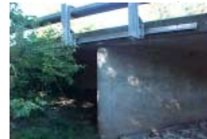
(f) Slab-Pier Connection
