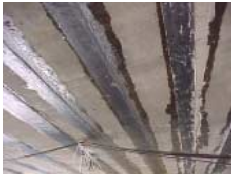
(a) Bonded CFRP Plates
