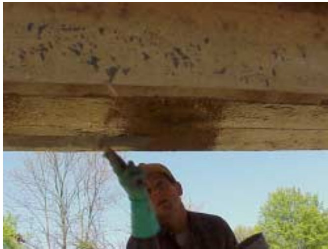
Application of Structural Epoxy on Primed Surface
