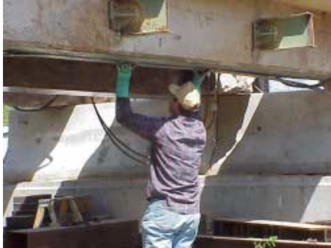
Installation of FRP plate
