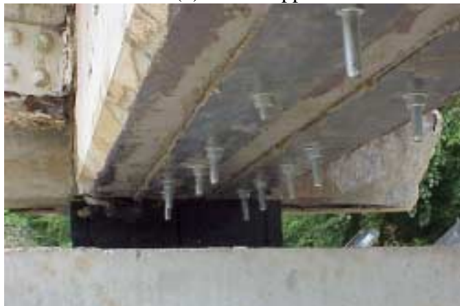
(c) Overall View of Bolts
