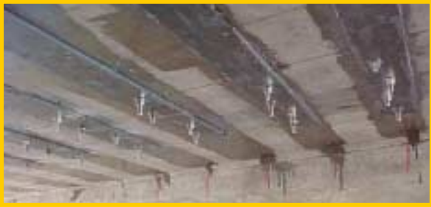
(b) Bolted CFRP Plates
