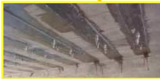
(b) Bolted CFRP Plates
