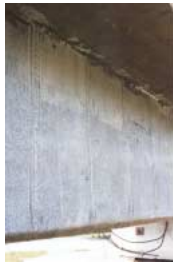
(c) View of Web Reinforcement
