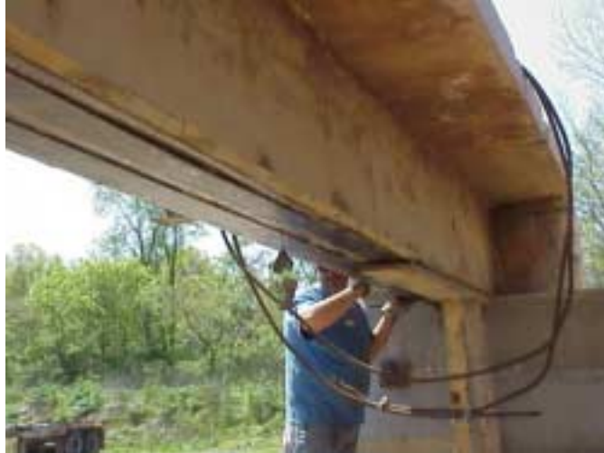
Shoring of 102-mm FRP Plates
