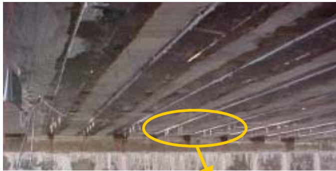
(a) Bonded CFRP Plates
