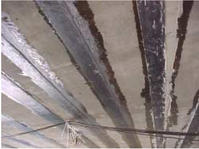
(a) Bonded CFRP Plates
