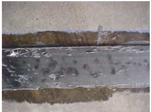
(e) Close-up view of FRP shortly after installation
