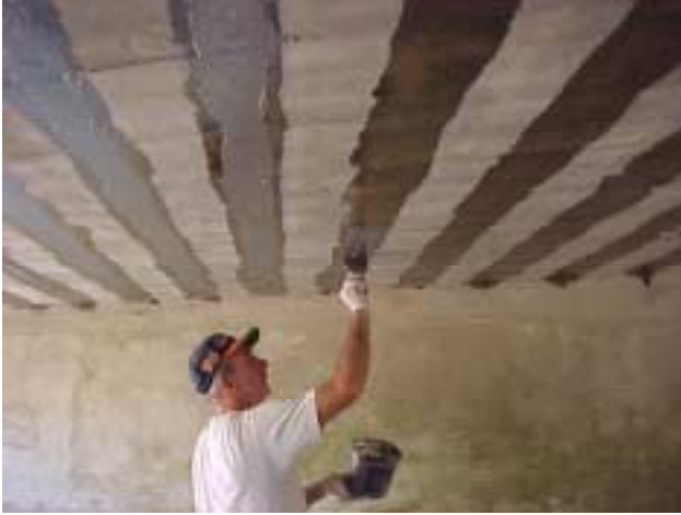
(a) Application of structural epoxy on primed surface
