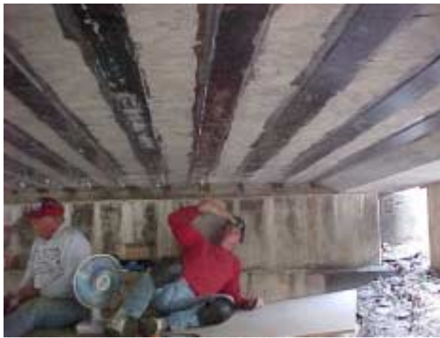
(h) Driving anchors into slab
