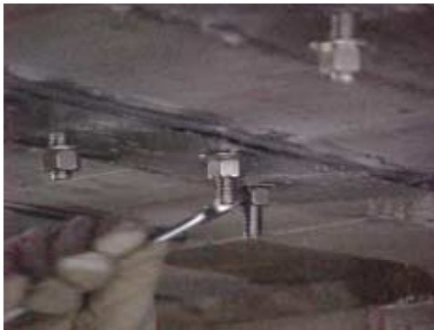
(i) Tightening of anchors
