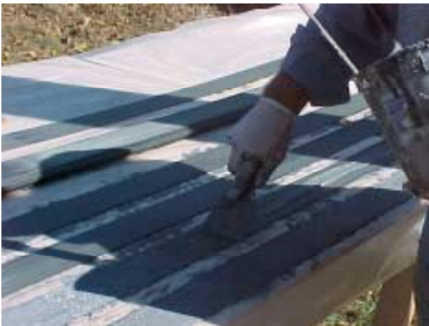
(c) Application of structural epoxy on cleaned FRP plates
