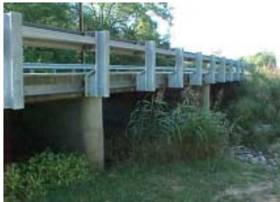
(e) Overall View of Bridge
