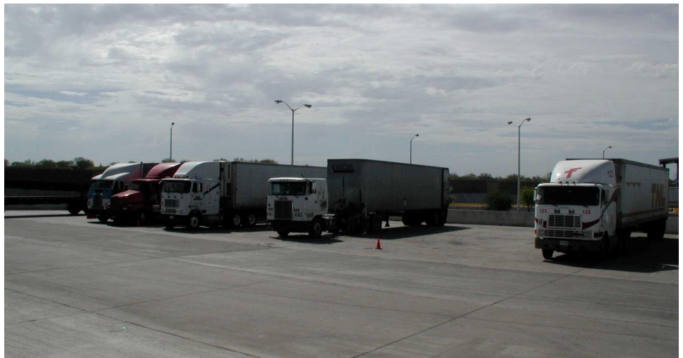
Figure 2: Truck Inspection Space at the World Trade Bridge, Laredo, Texas
