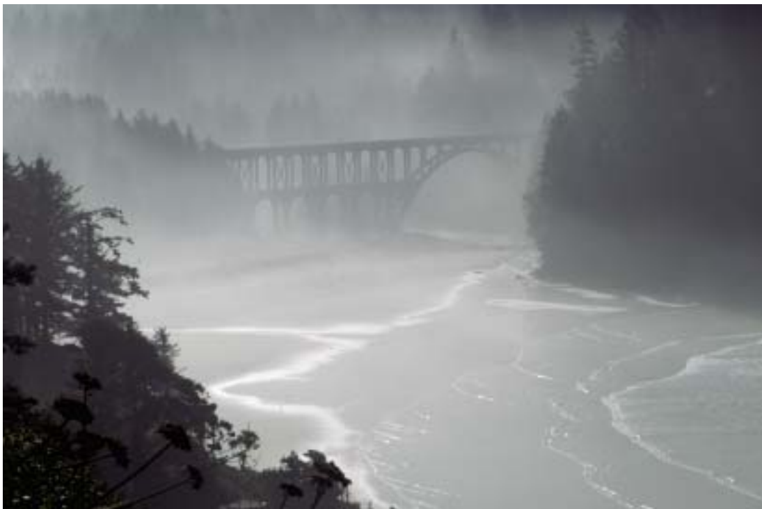
Figure 1.3: Cape Creek Bridge showing morning fog that aids the deposition of salt on the bridge surface as a precursor to chloride-induced corrosion damage
