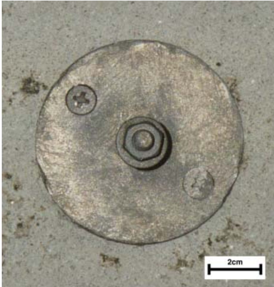
Figure E.1: Terminal plate connection prior to thermal spraying with Zn
