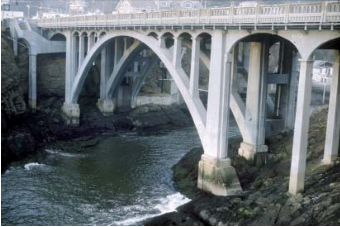
Figure 1.6: Depoe Bay Bridge built in 1927, widened in 1940, and located on the Oregon coast at Depoe Bay
