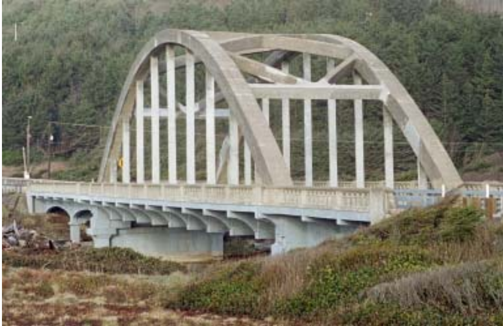
Figure 1.8: Big Creek Bridge built in 1931 and located on the Oregon coast south of Cape Perpetua
