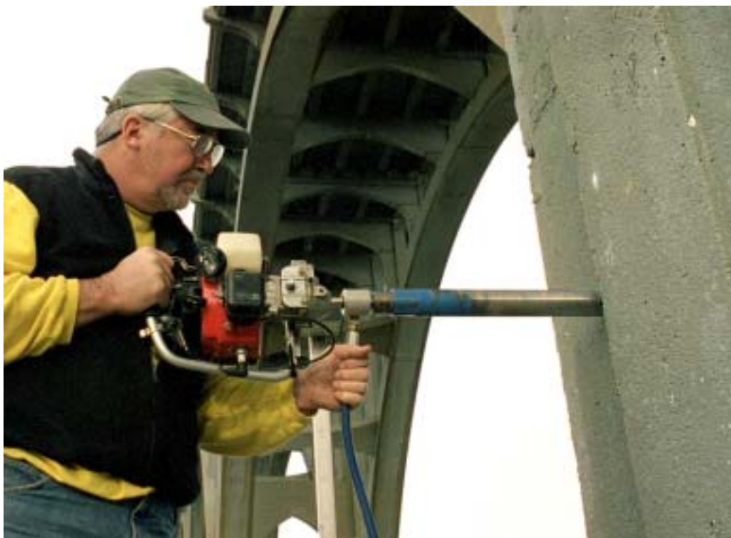
Figure 3.11: Portable gasoline-powered core drill for taking concrete core samples
