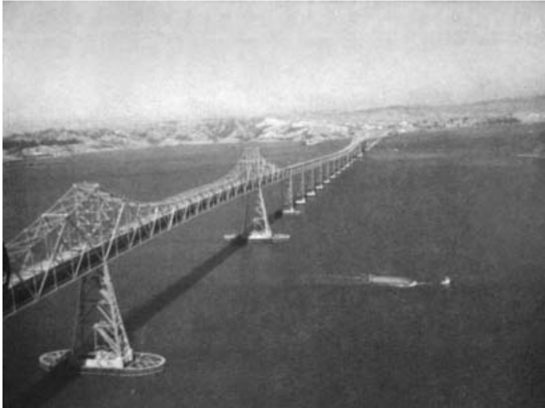
Figure 2.9: Richmond-San Rafael Bridge (CA) built in 1956 spans the northern San Francisco Bay
