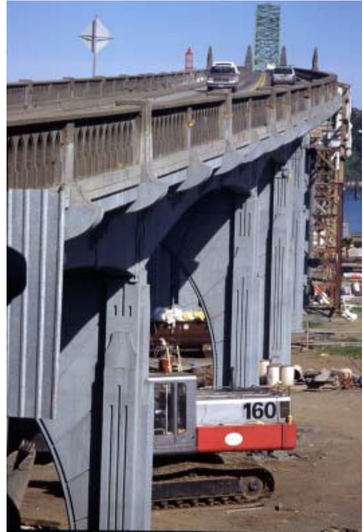
Figure 1.5: South approach of the Yaquina Bay Bridge
