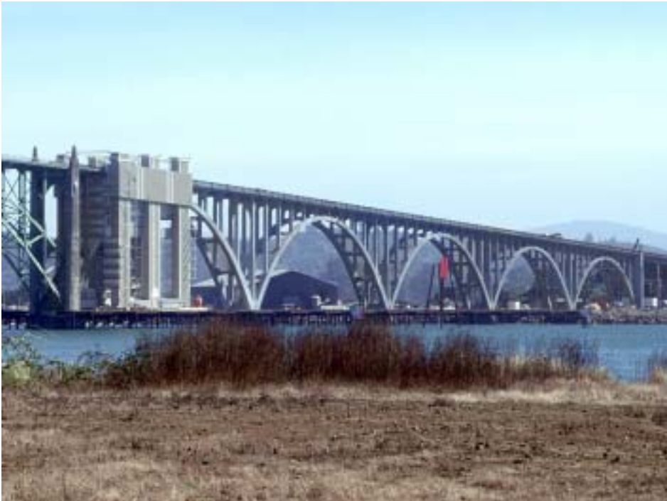
Figure 1.4: Yaquina Bay Bridge built in 1936 and located on the Oregon coast at Newport
