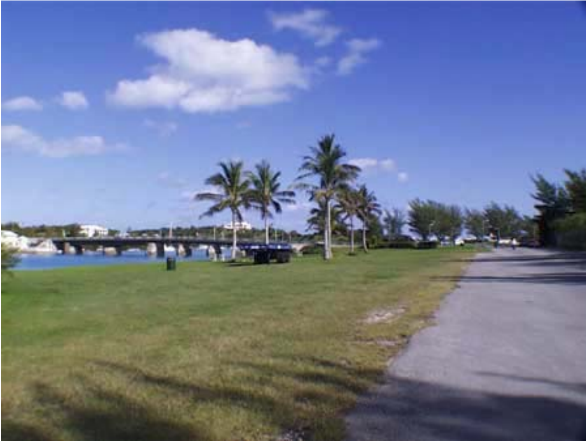
Figure 2.14: Longbird Bridge built in 1948 in Bermuda
